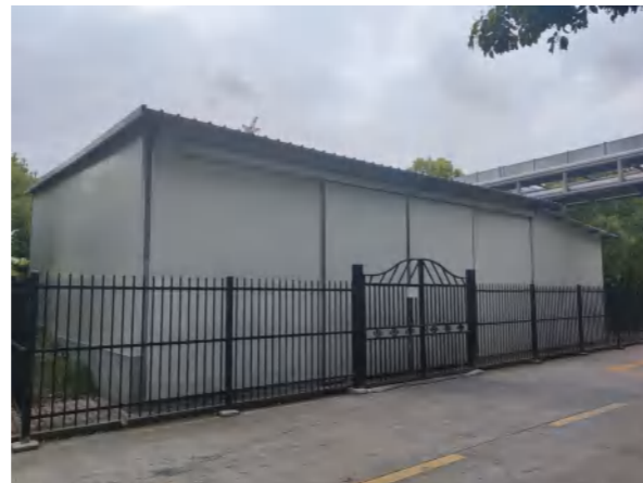
Wastewater treatment pool
