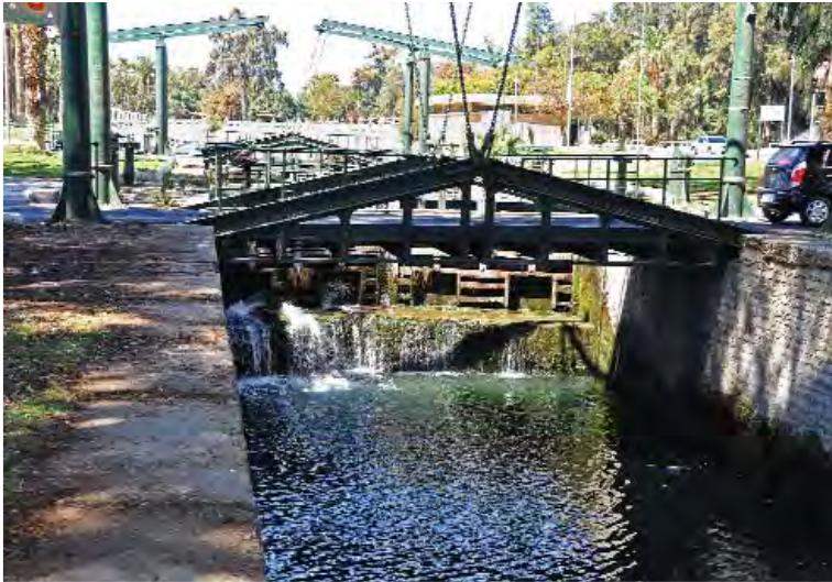
Left: The Ismailia Canal is slightly higher than Lake Timsah where it enters the lake. Sluice-gates prevent salty water from flowing back into the canal, whose water is used for the irrigation of fields cultivated for agriculture.
