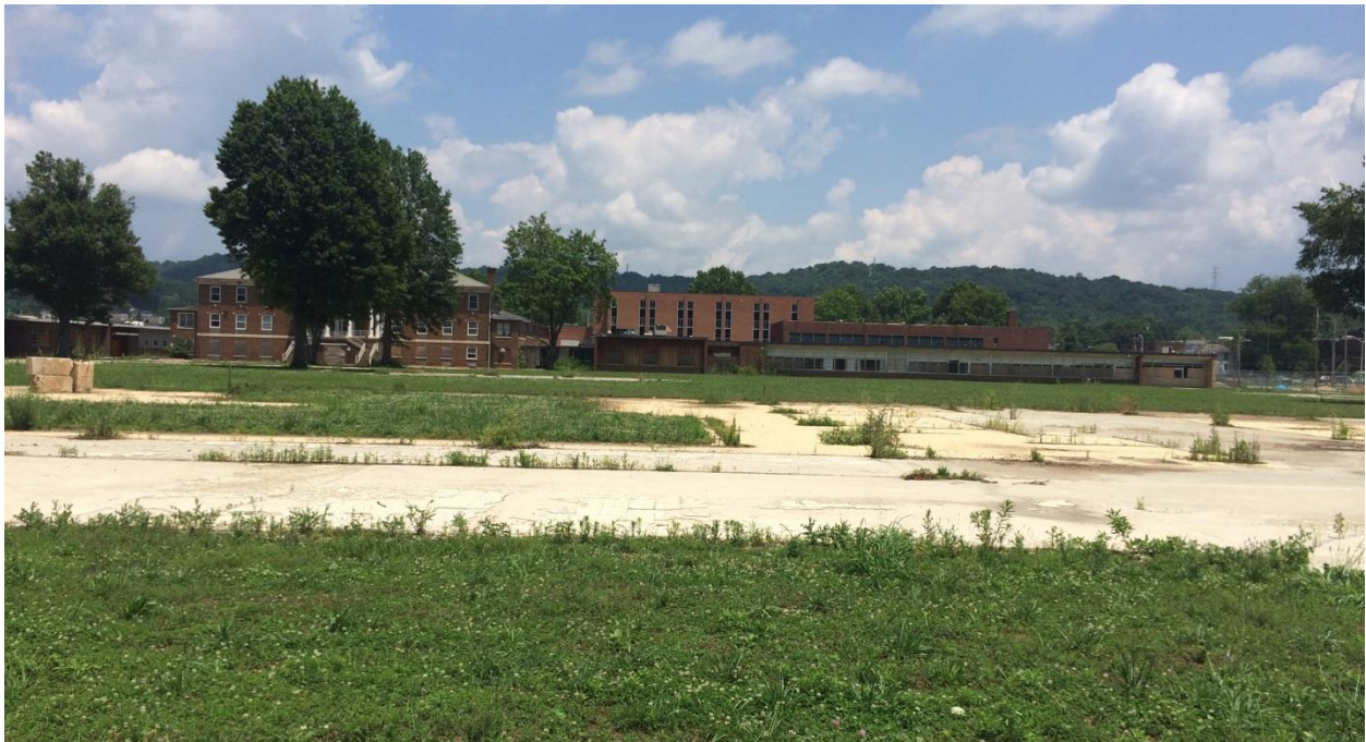
Center of Subject Property Facing North Toward Former Building C of Rehabilitation Center (Photo 10)
