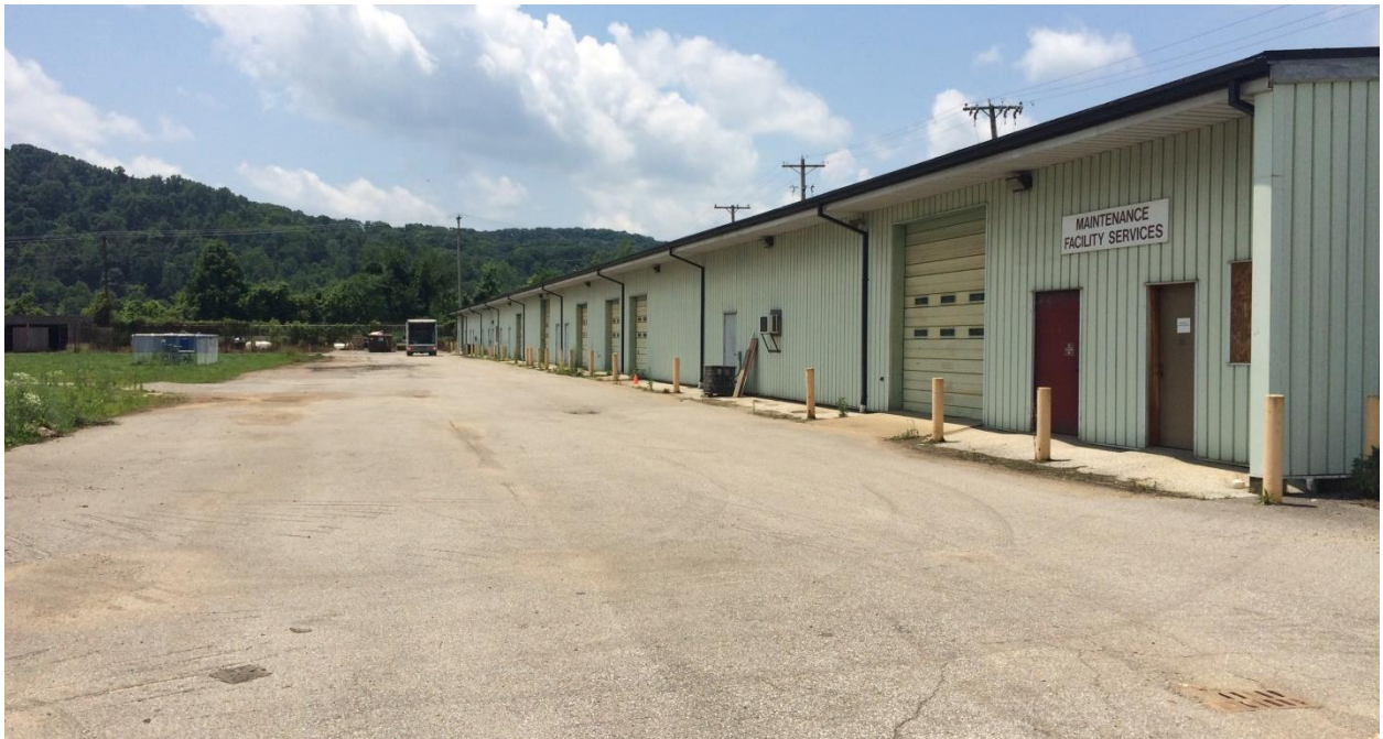
Southwestern Extent of Subject Property Maintenance Facility Facing South (Photo 12)
