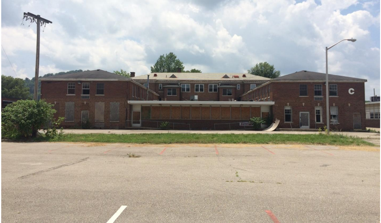
Rear of Building C Facing South (Photo 17)
