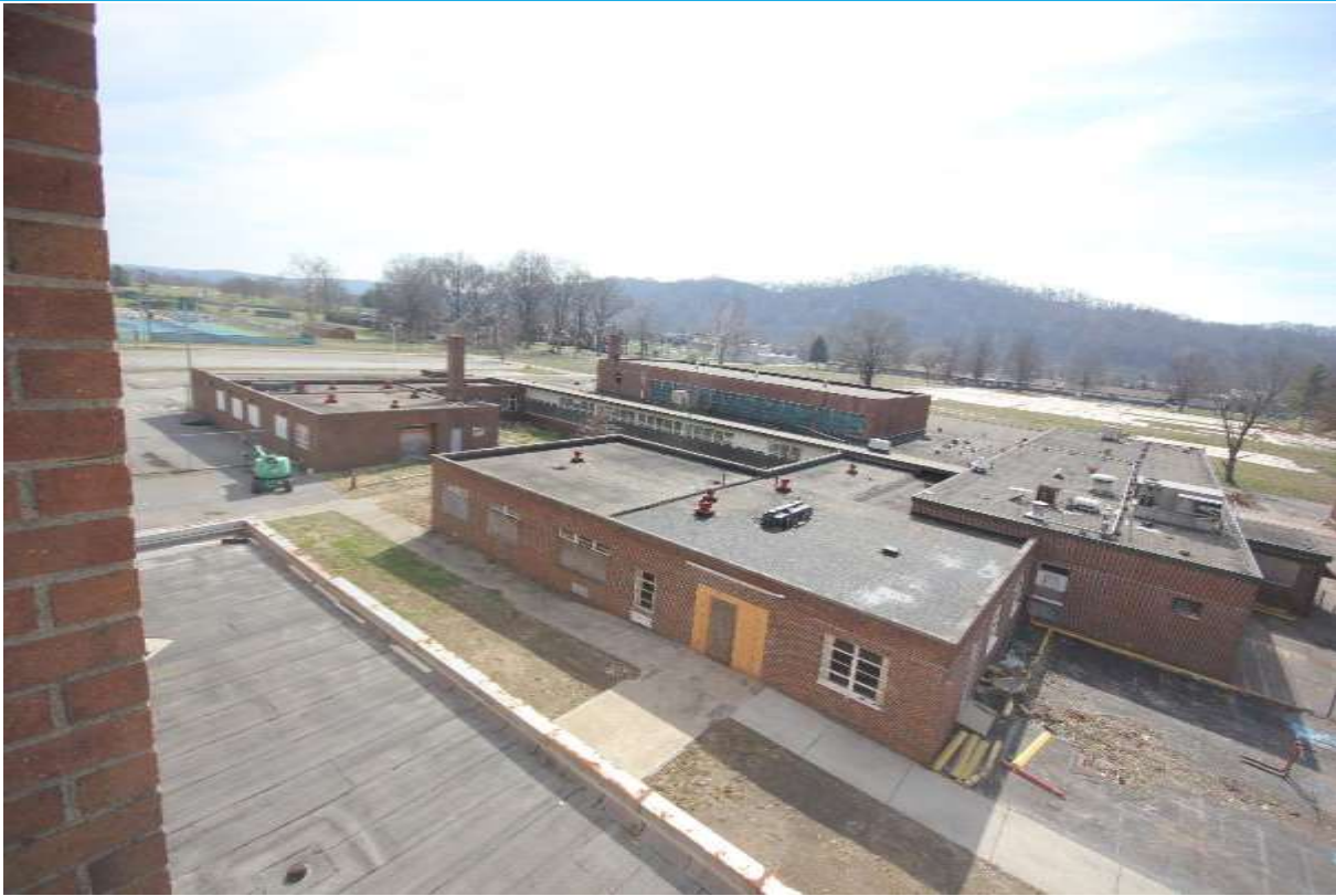
4. WV School for the Colored Deaf and Blind Gymnasium, looking southeast from F. Ray Power Building
