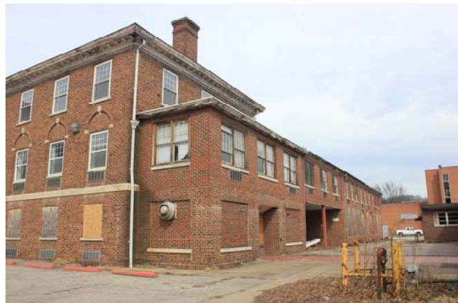
East Wing looking north.
