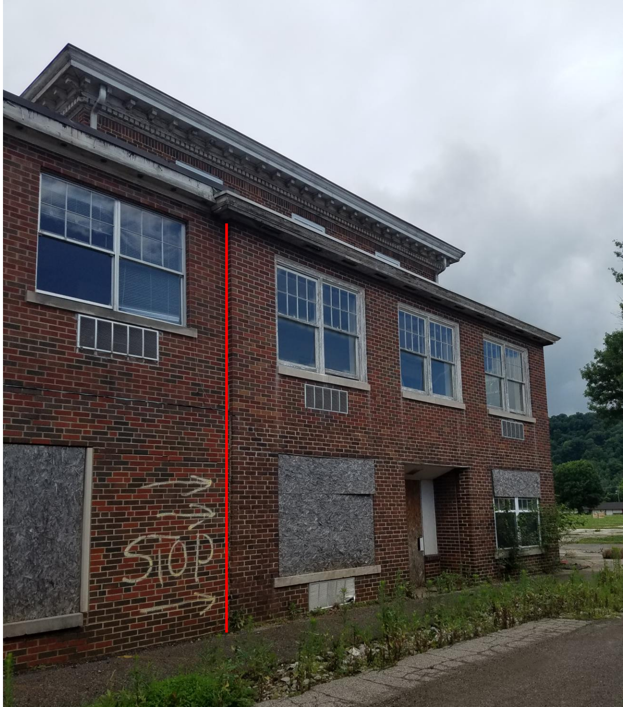
West Side of Building C Displaying Original Building and West Wing Corridor Extension (Photo 27)
