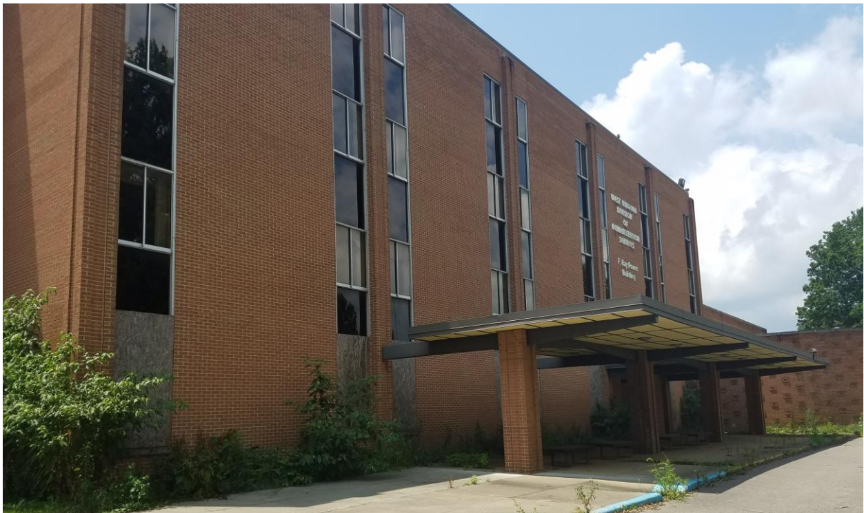
Front of F. Ray Powers Building Facing Southwest (Photo 20)
