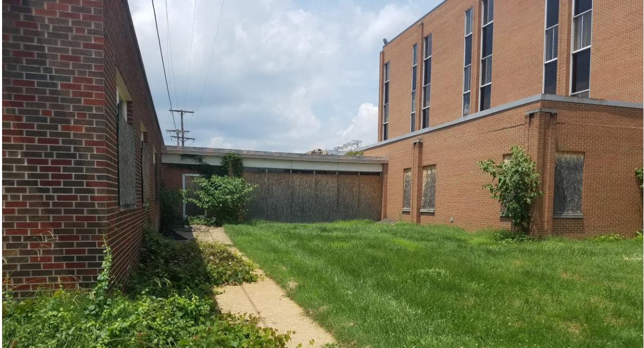
Corridor connecting F. Ray Powers Building to East Wing of Building C (Photo 21)
