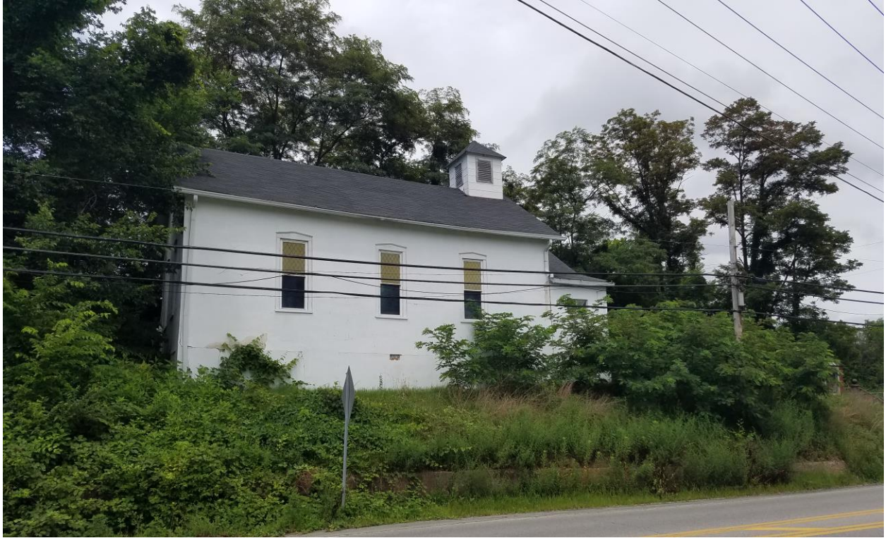
Samaritan Baptist Church Facing Northeast (Photo 31)
