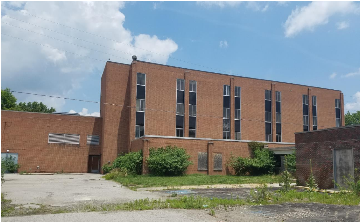
Rear of Building C Facing Northeast (Photo 18)
