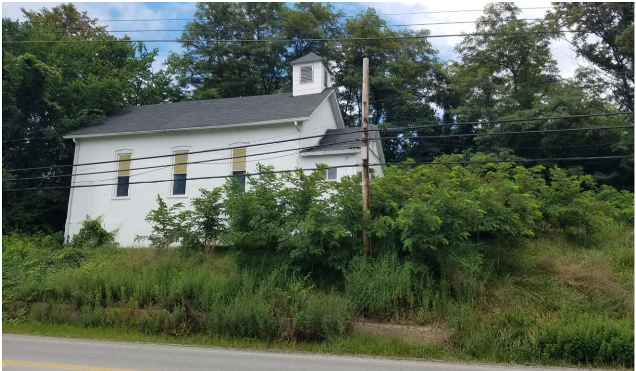
Samaritan Baptist Church Facing Northwest (Photo 32)
