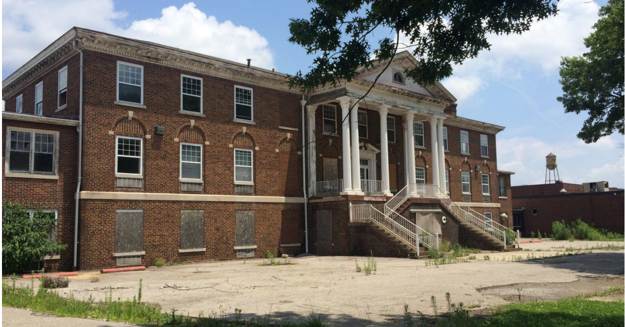
Front of Building C Facing Northeast (Photo 13)
