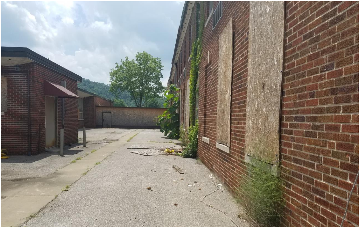
Area in Between Building C East Wing Facing South (Photo 16)
