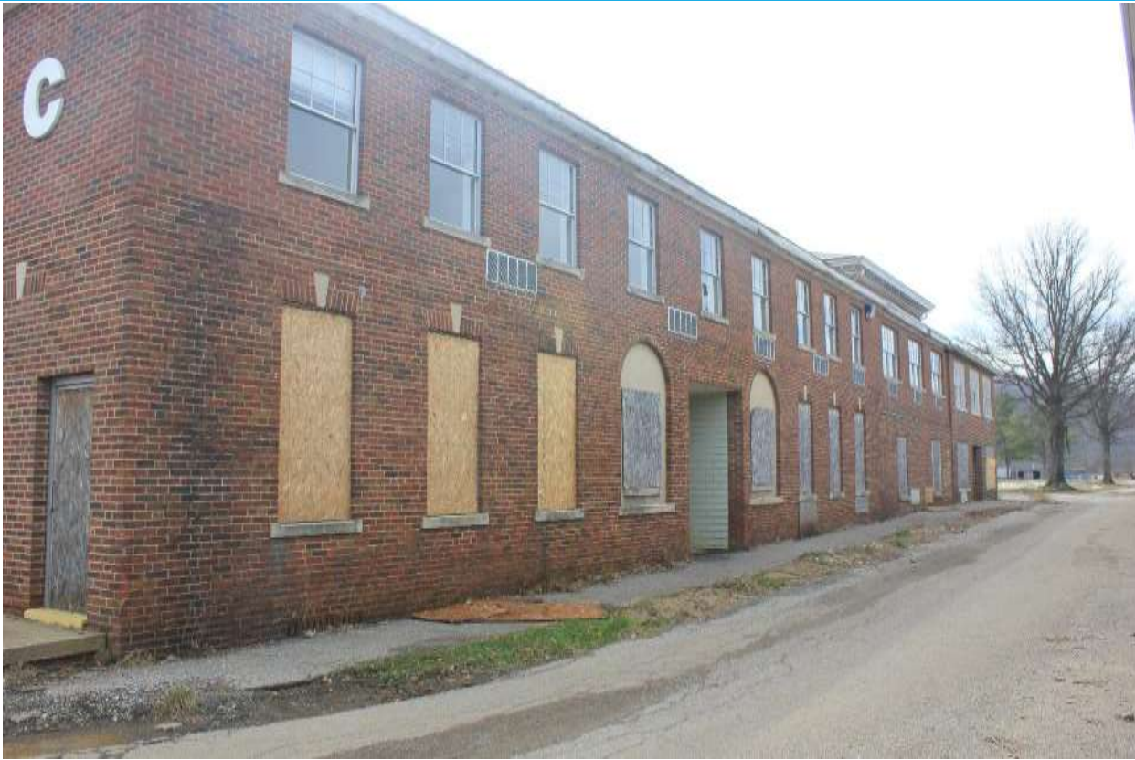
8. WV School for Colored Deaf and Blind west wing, looking south
