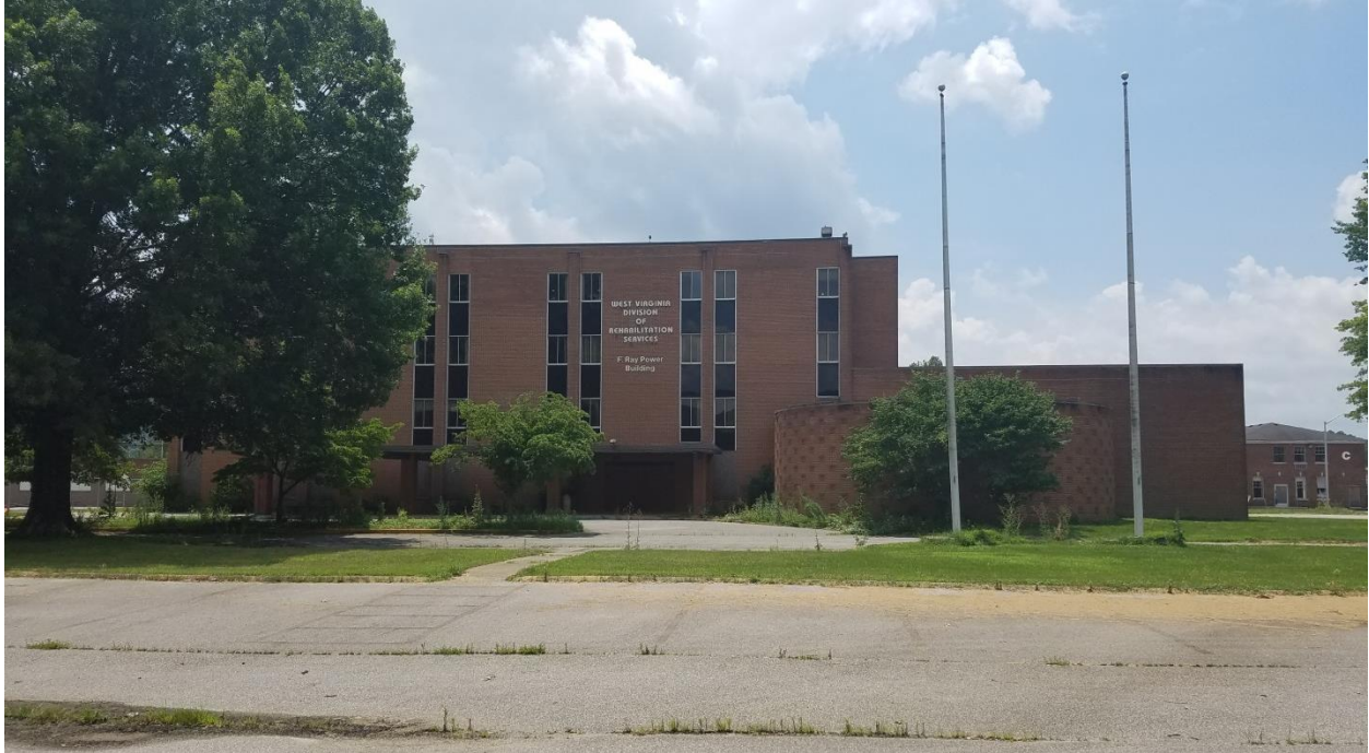
North (Front) of F. Ray Powers Building Facing South (Photo 19)
