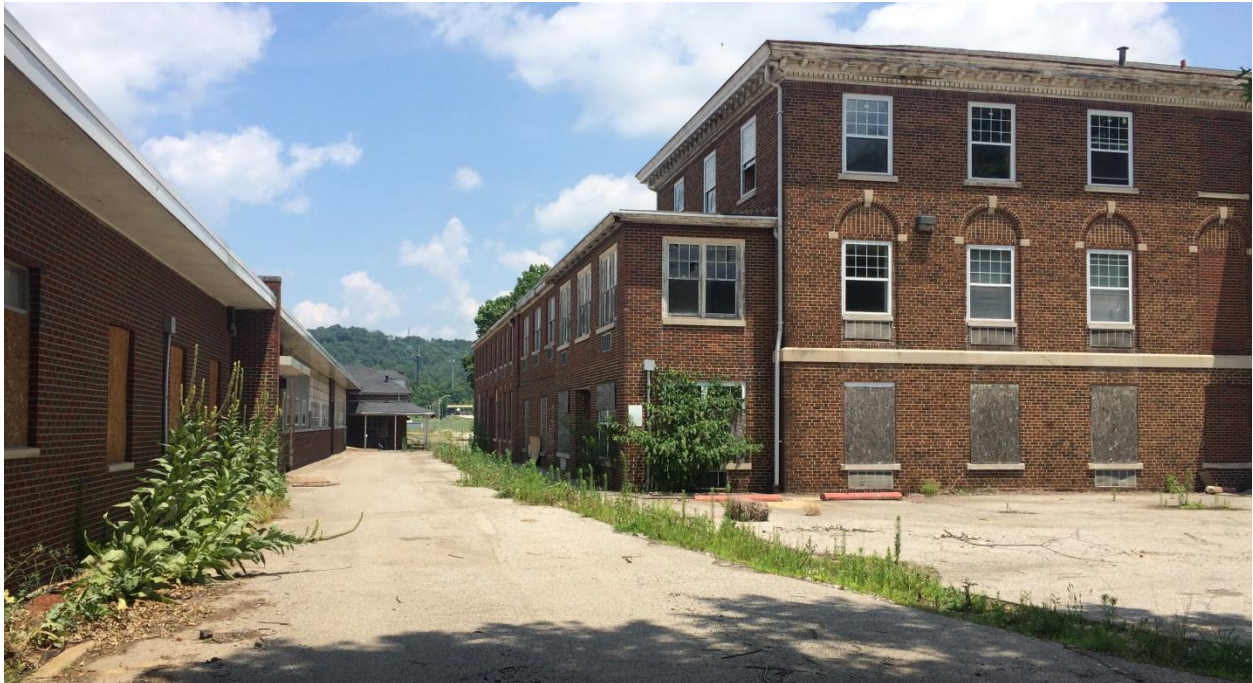
Front of Building C and Building E Facing North (Photo 14)
