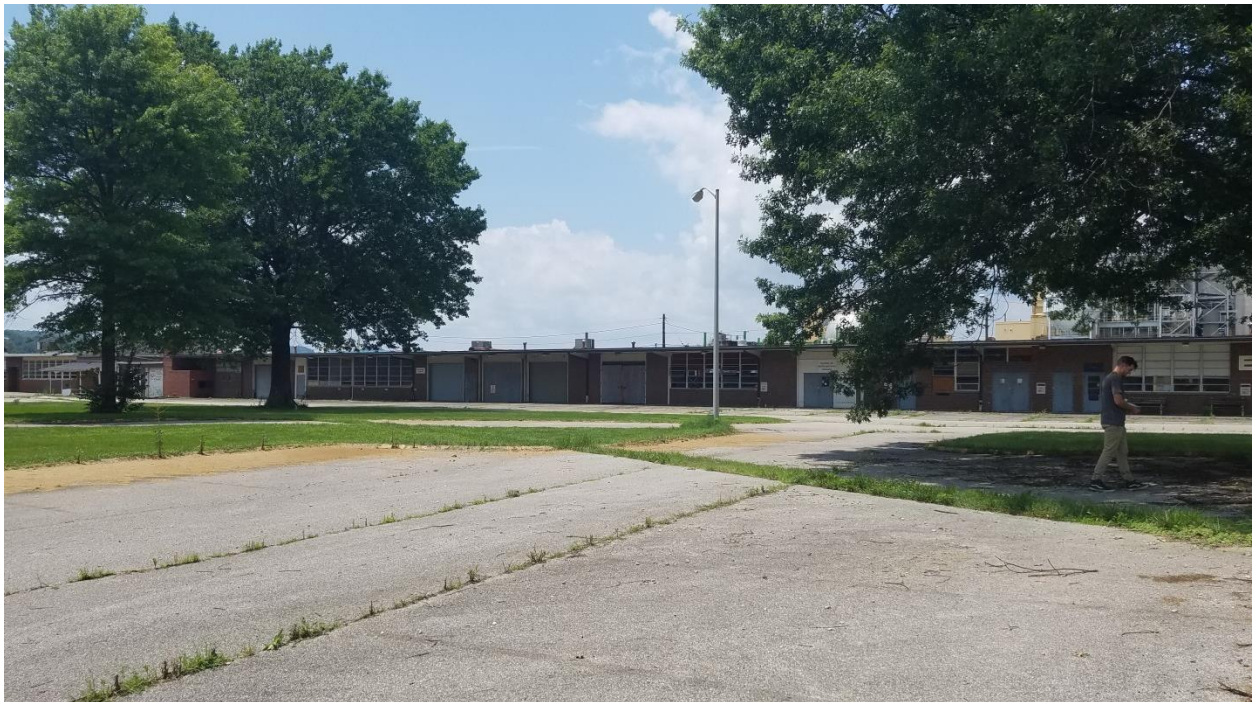
Front of Building E Facing Southwest (Photo 22)
