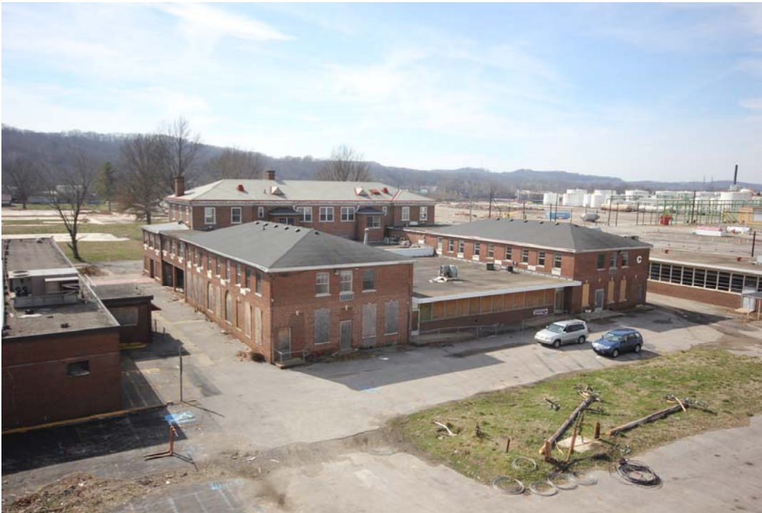
Overview looking south from F. Ray Power Building.
