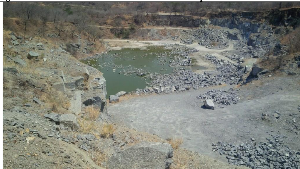
View of the Existing Disused Sinhydro Quarry (Preferred Waste Rock Dump Site)
