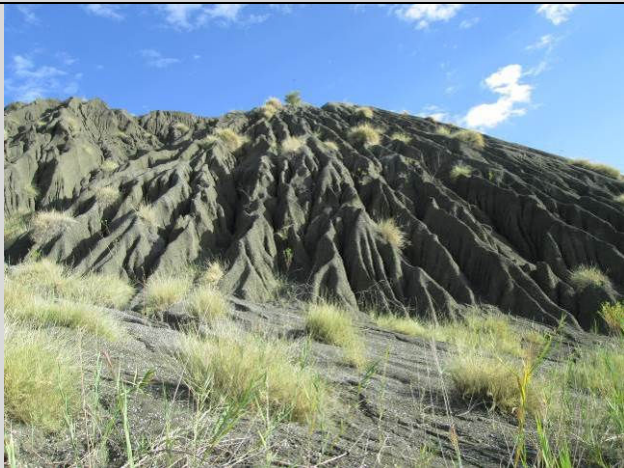
Evidence of erosion off the Slimes dam
