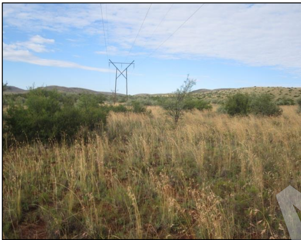
Figure 6: Vegetation growing under medium-sized power lines
