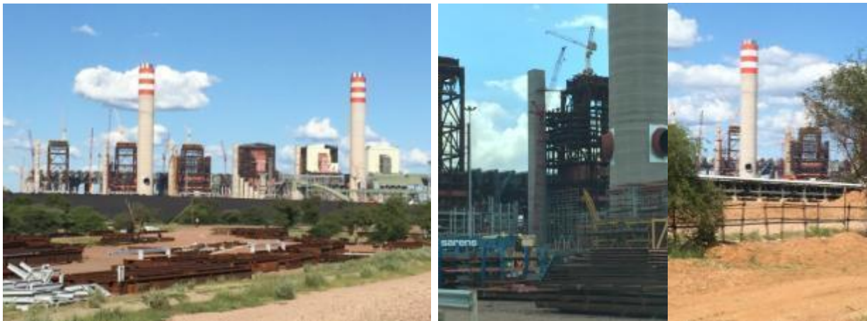
Ongoing construction of the MPS
