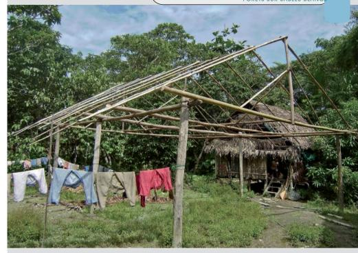
Photograph 2. Wooden house structure made with small diameter round wood coming from white-sand forests. Photograph R. de Oñate.
