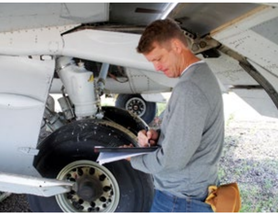
Above: F/O Leon Petruccio (Delta) takes detailed notes to document the condition of the landing gear, gear doors, nearby structure, and tires.
