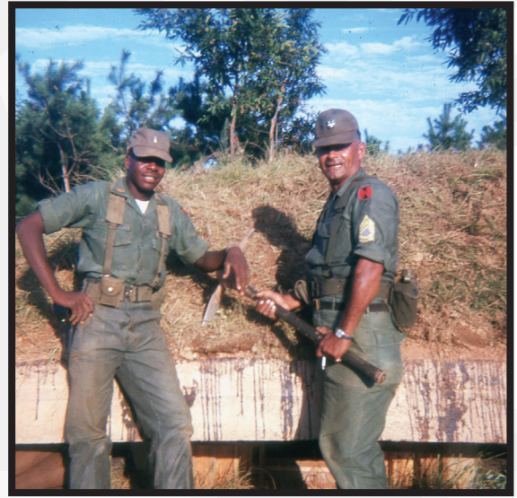
Working on "Phase Line Papa" 1968 Lt Jurwood Moxley and 1SG Ramirez
