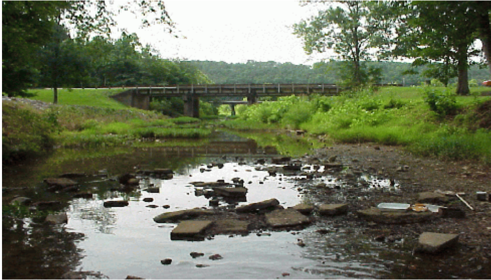
Station CR-AT: Downstream
