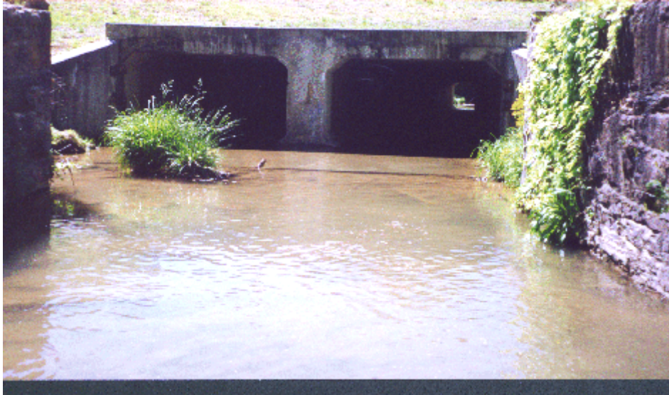
Station UT-1: Downstream
