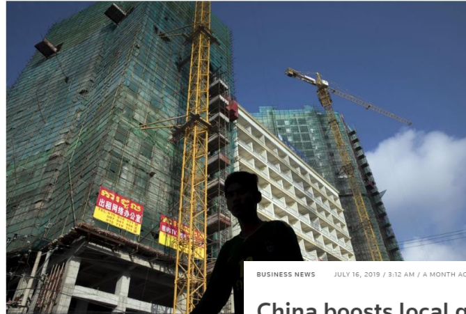
ion site in Sihanoukville, Cambodia
