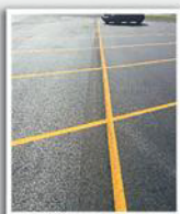
FIGURE 1 Rogers, Arkansas: SmartMIX parking lot application.
