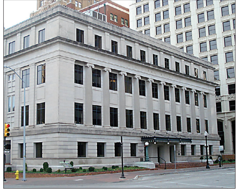
Courtesy photo MUNICIPAL BUILDING: The Tulsa Municipal Building at 124 East 4th St. was built in 1917 and served as Tulsa's City Hall until 1969. It sat vacant for four years until it was restored to professional office occupancy. It is listed on the National Register of Historic Places.
