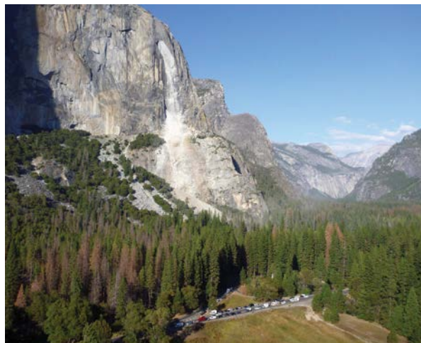
Rockfall on the right side of El Capitan in September 2017. The Waterfall Route, located in this area, has continued to shed rock in 2018. NPS Photo
