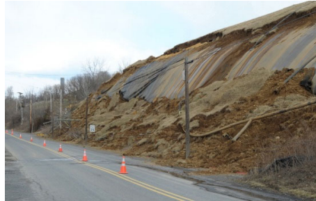
Figure 4: Translational Failure at a landfill site
