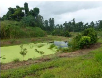
Polishing ponds are the ultimate in water filtration. Waste water from the packing shed passes through a series of settling ponds that remove organic and waste material, before the water is discharged.
