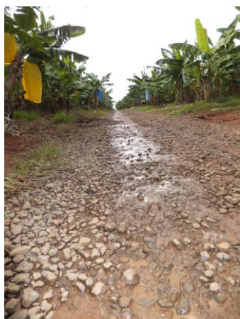
Stabilise areas with rock to reduce sediment movement.
