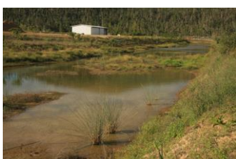
This constructed wetland helps to remove suspended solids from runoff water before it leaves the banana farm.
