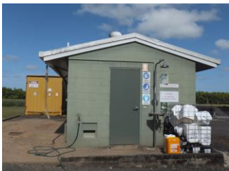
Store chemical containers in a suitable location until disposed of.
