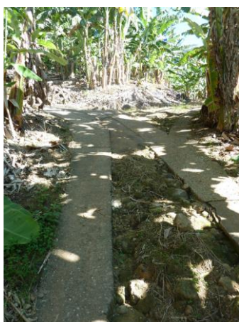
Concrete roadways provide all weather access in steeper areas, for example on the subtropics east coast.
