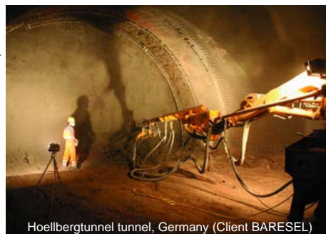
Hoellberg tunnel, Germany (Client BARESEL)
