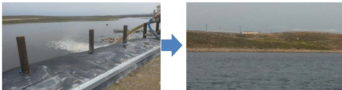
Figure 45. Wastewater in Cambridge Bay is treated in a lagoon-tundra wetland system, and then discharged into the bay.
