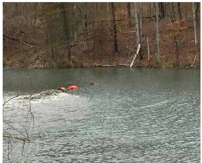
Figure 3. Dredging and depositing ash. Left photo: dredge near the cut area in the ash delta. Right photo: discharge pipe in the ash basin finger adjacent to the landfill.
