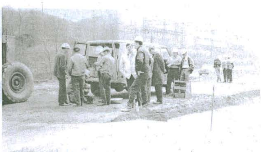
West Virginia State highway officials and a number of interested roadbuilders viewed the Rt. 2 project with a great deal of interest.
