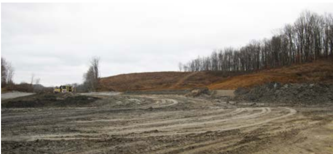
(6) Backfilling of highwall in December 2014.
