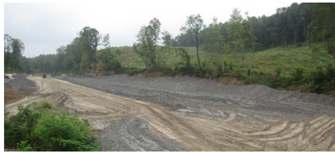
(5) Placement of sFGD and FGD gypsum in August 2013.
