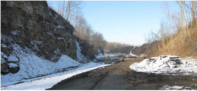
(3) Site preparation in February 2012.
