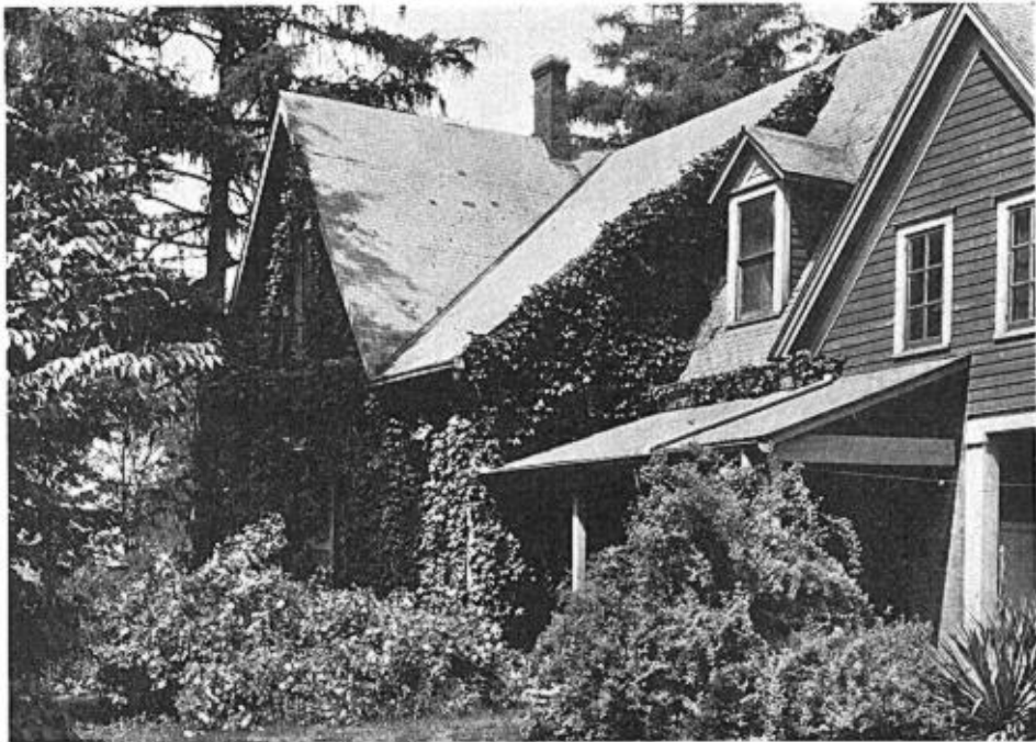
Fig. 46. THE RESIDENCE AT LARCHMOUND.
