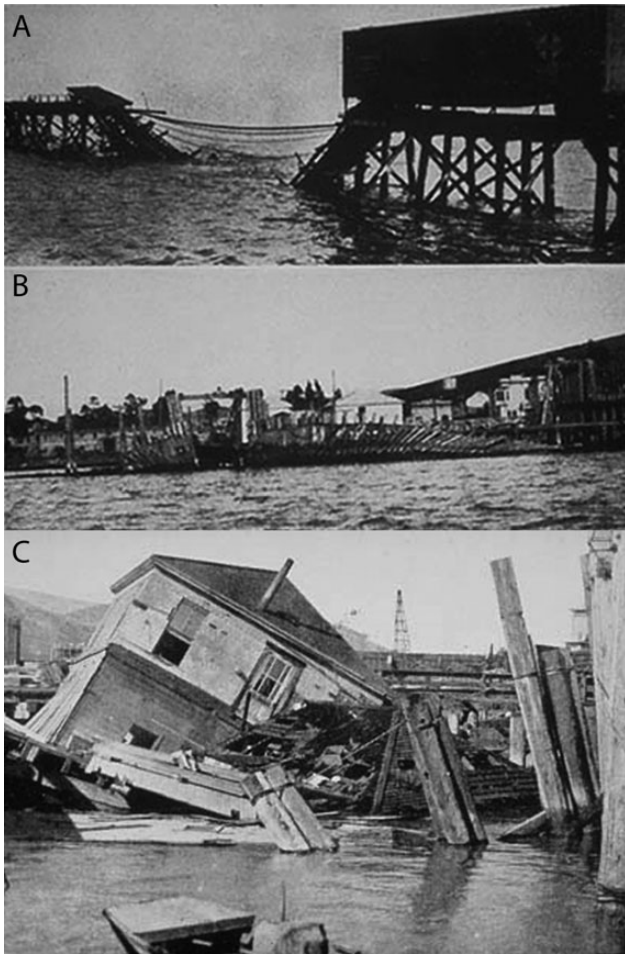
Figure 1. Destruction in the San Francisco Bay area attributed to Teredo navalis in three historical photographs. Photo: Union Oil Co. from Hill & Kofoid (1927).
