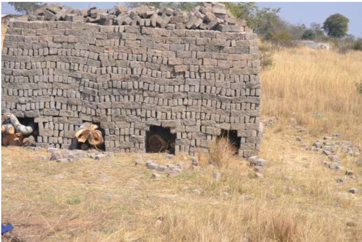
Figure 6. Example of a Kiln for baking moulded brick. Source: Author
