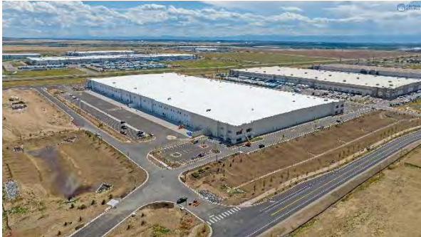
Aerial of Building E facing SW
