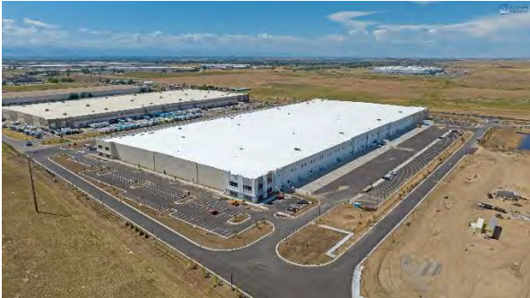
Aerial of Building E facing NW
