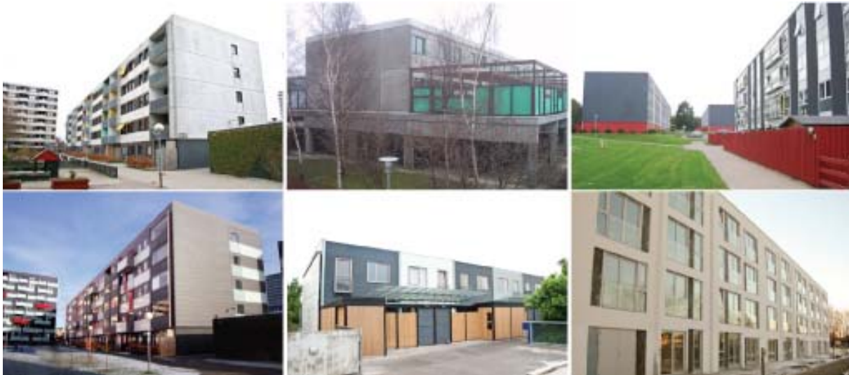
Figure 1: Case studies, before and after/during renovation
