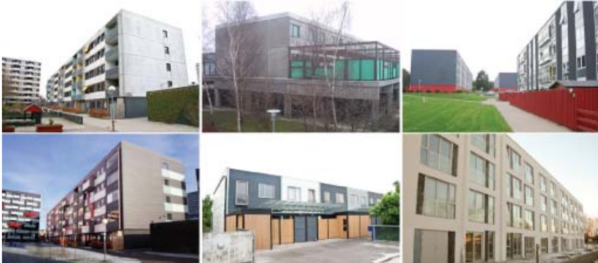
Figure 1: Case studies, before and after/during renovation
