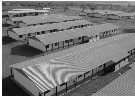
Figure 4. View of temporary constructions in cellular concrete. Source: http://www.prefacc.com.br/
