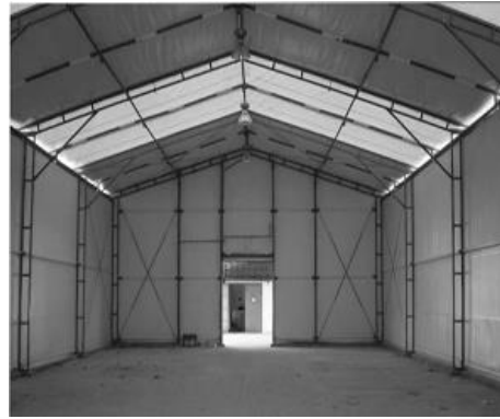
Figure 14. Shed, without internal pillars Source: http://www.sansuy.com
