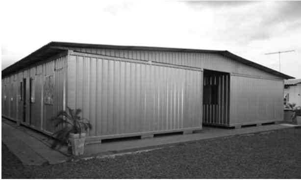
Figure 9. Temporary facilities in galvanized steel. Source: http://cmcmódulos.com.br
