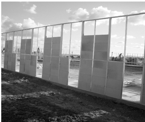
Figure 3. Assembly of temporary facilities in cellular concrete. Source: http://www.novoespaco.com.br
