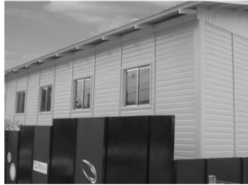
Figure 2. Prefabricated temporary facilities made with pinewood panels. Source: http://www.canteiro.com.br/
