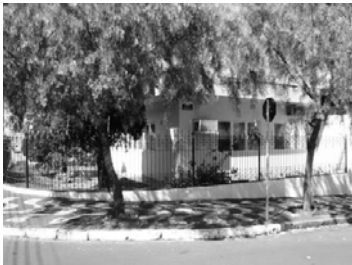
Figure 10. Windows of a building in Araras, which provide cross ventilation.
