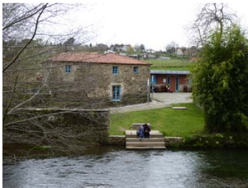
Figure 15. General view of the hostel next to the river.
