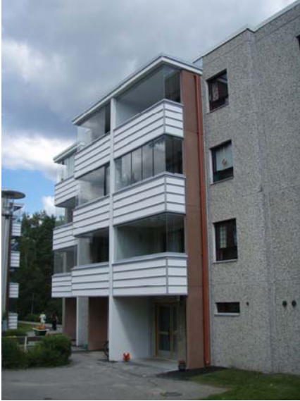
Figure 1. Typical Finnish concrete balcony with balcony glazing.
