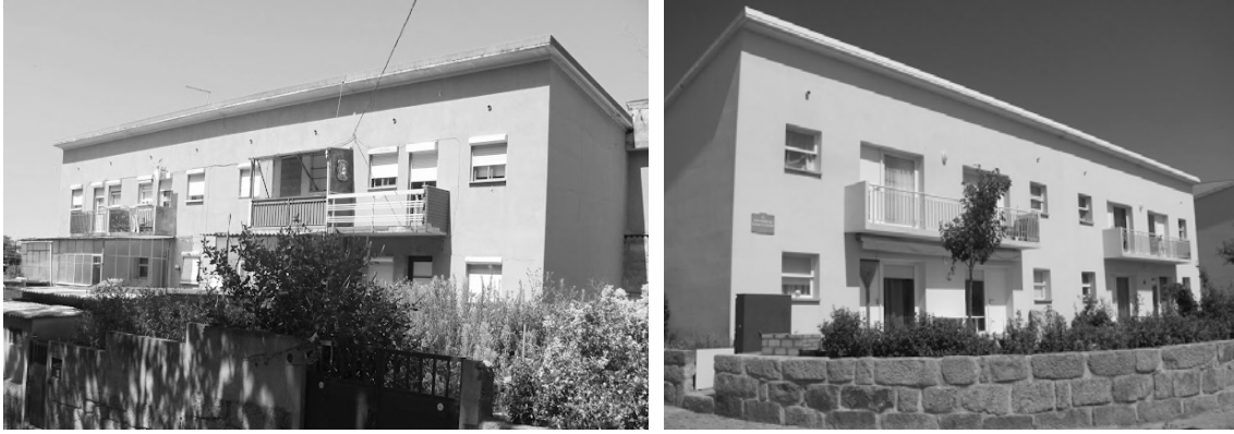
Figure 1 Building before and after renovation on Rainha Dona Leonor neighborhood
