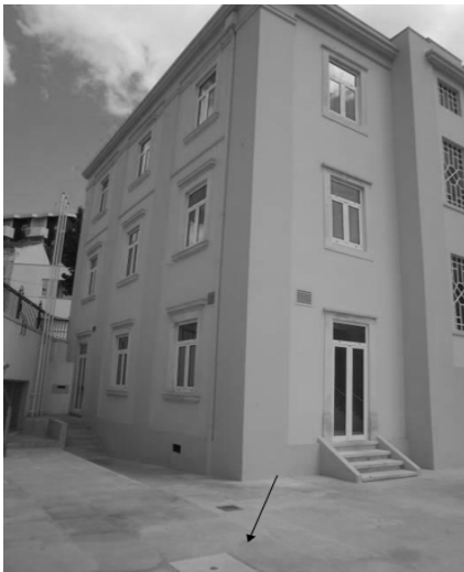
Figure 2. The water storage tank under the floor terrace
