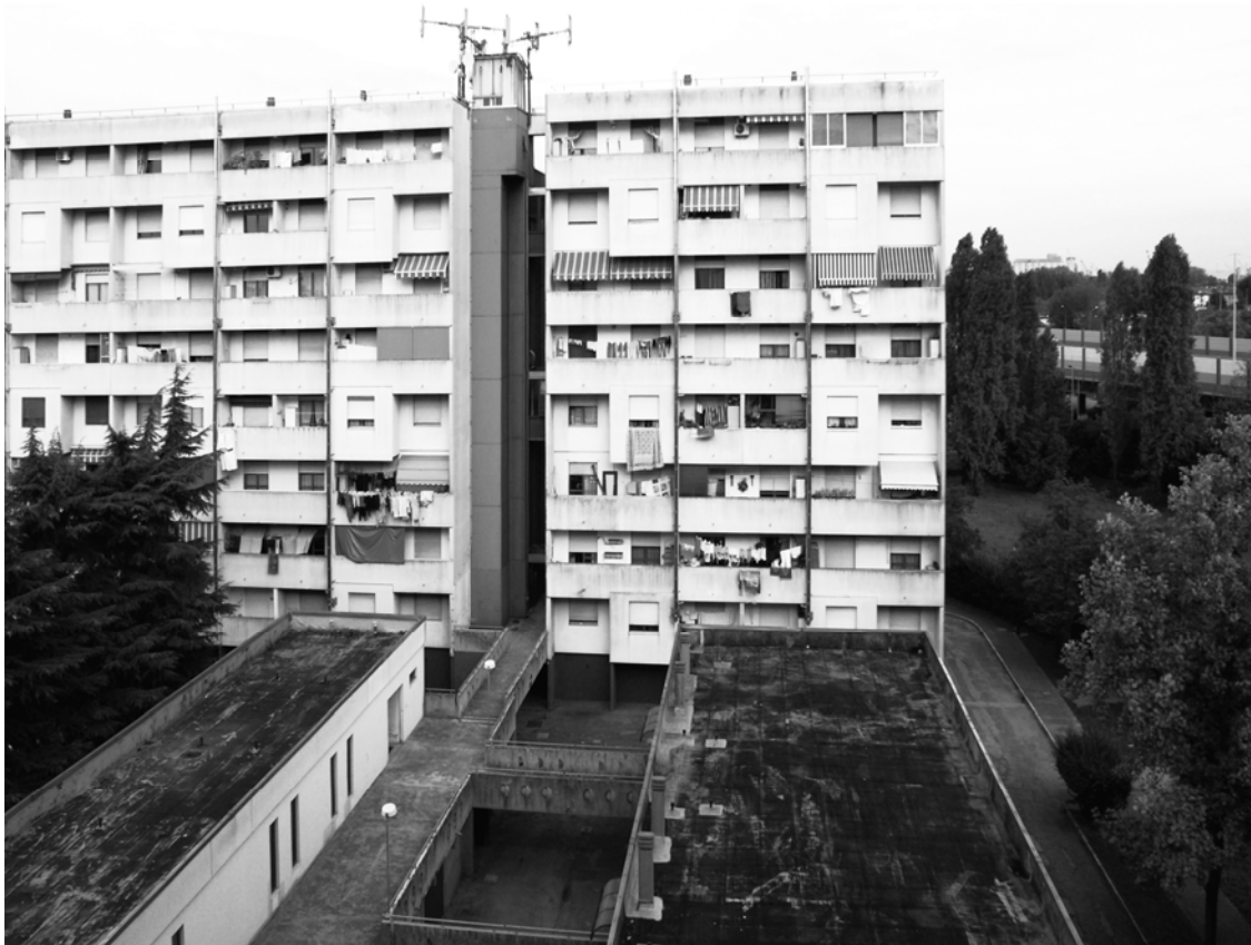
Figure 2. The social housing compound in via Bosco, Marghera (Venice)
