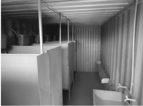
Figure 5. Internal detail of a container used as a bathroom.
