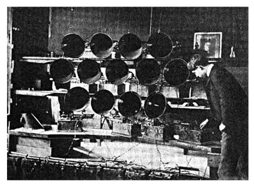
A bank of thirteen recording machines in the Edison studio. Setups like these were used in recording by the "round" method, with each machine yielding a master that would be used to pantograph individual copies for sale. Masters typically wore out after a few dozen playings, requiring frequent remakes. (*The Leisure Hour*, 1902–1903 Edition)
