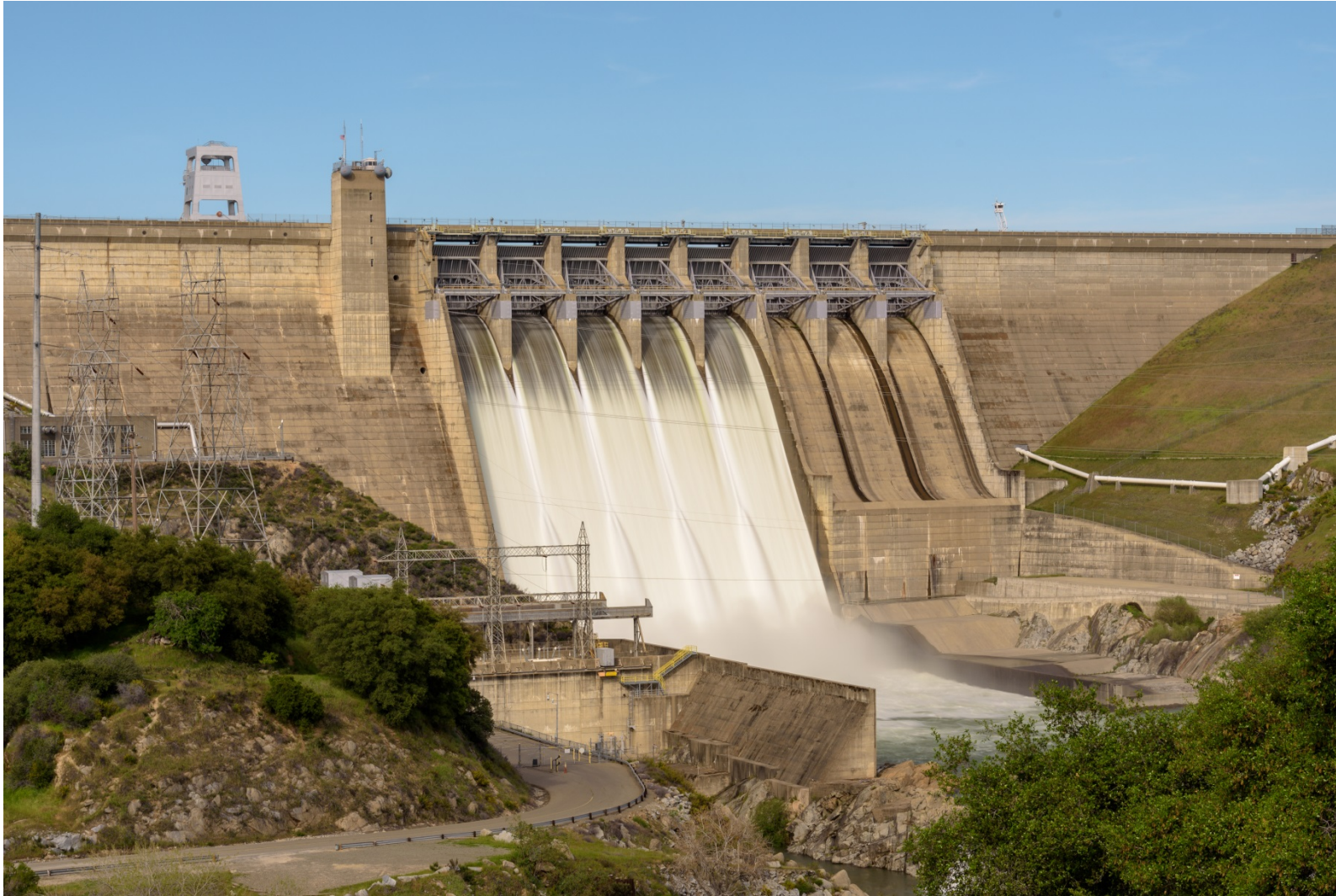
Figure 122. Folsom Dam (Source: image courtesy of William A. Fraser).
