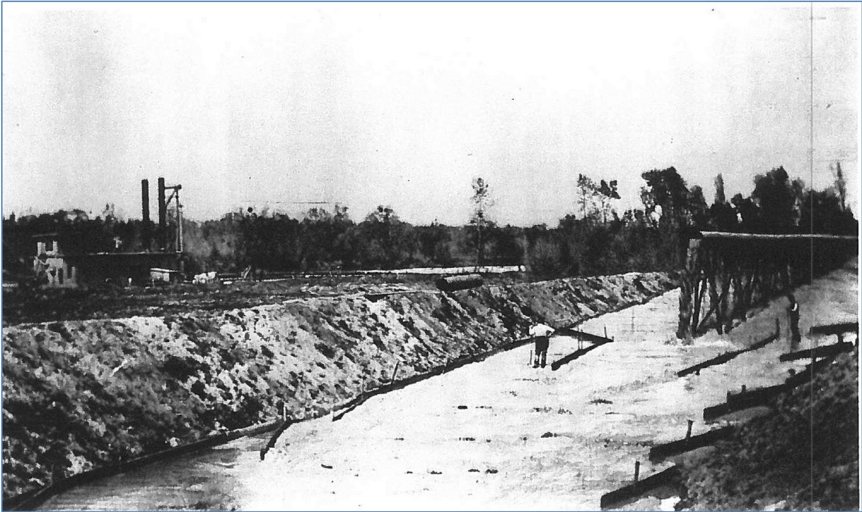
Figure 128. Suction dredge. Discharge is along right hand side of photograph. (Source – California Department of Water Resources).
