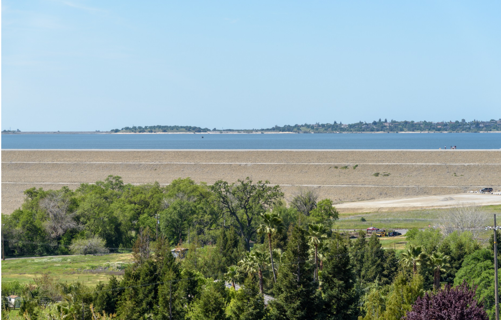
Figure 123. Left (eastern) portion of the Mormon Island Auxiliary Dam (Source: image courtesy of William A. Fraser).
