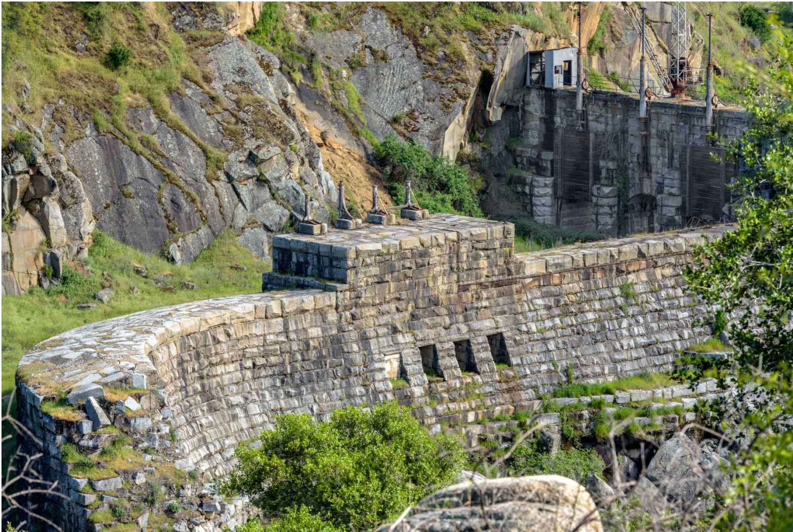
Figure 120. Remnant of Folsom Prison Dam (Source: image courtesy of William A. Fraser).
