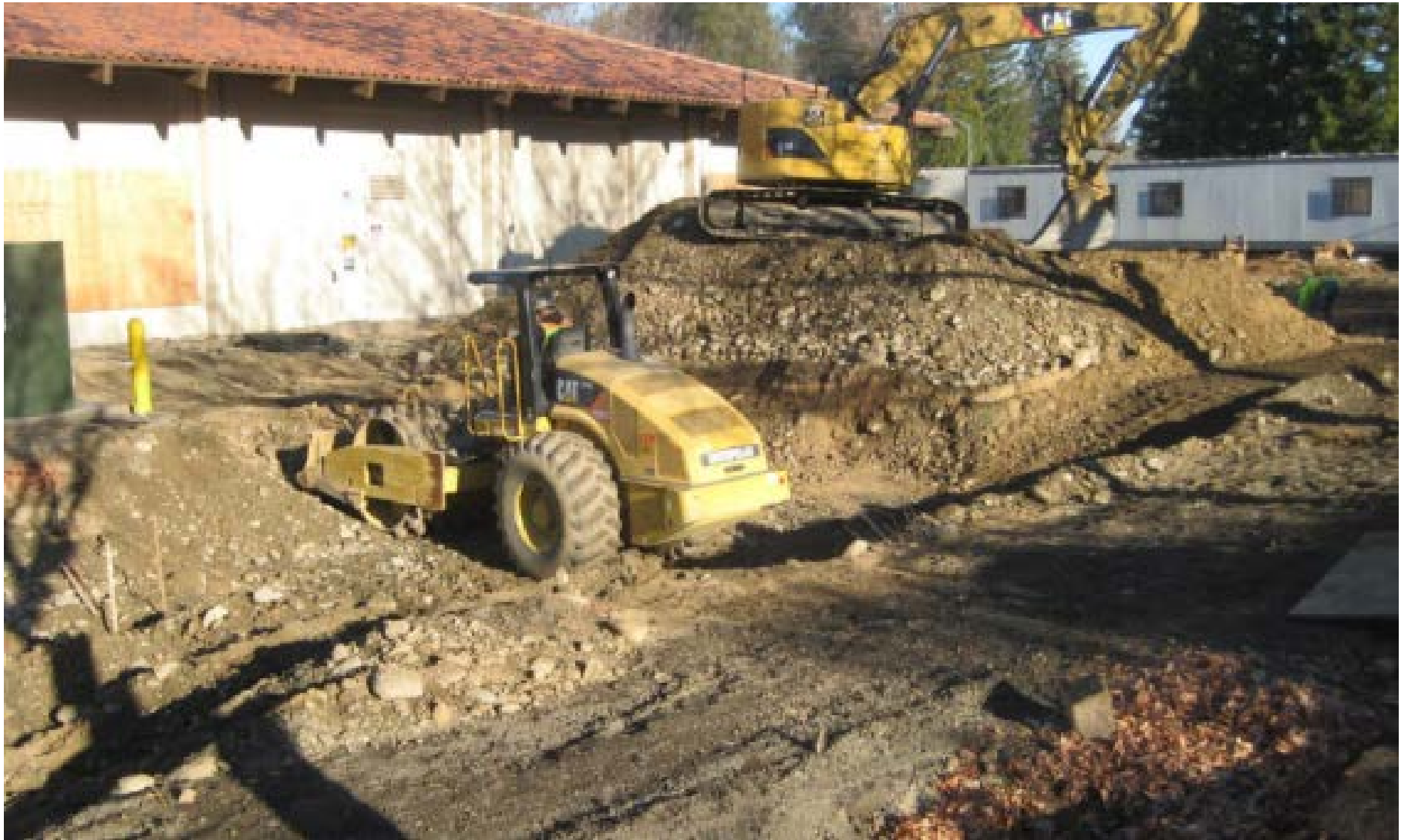
Figure 109. Photograph of remedial grading in dredge tailings (Source: image courtesy of Jeremy Zorne).
