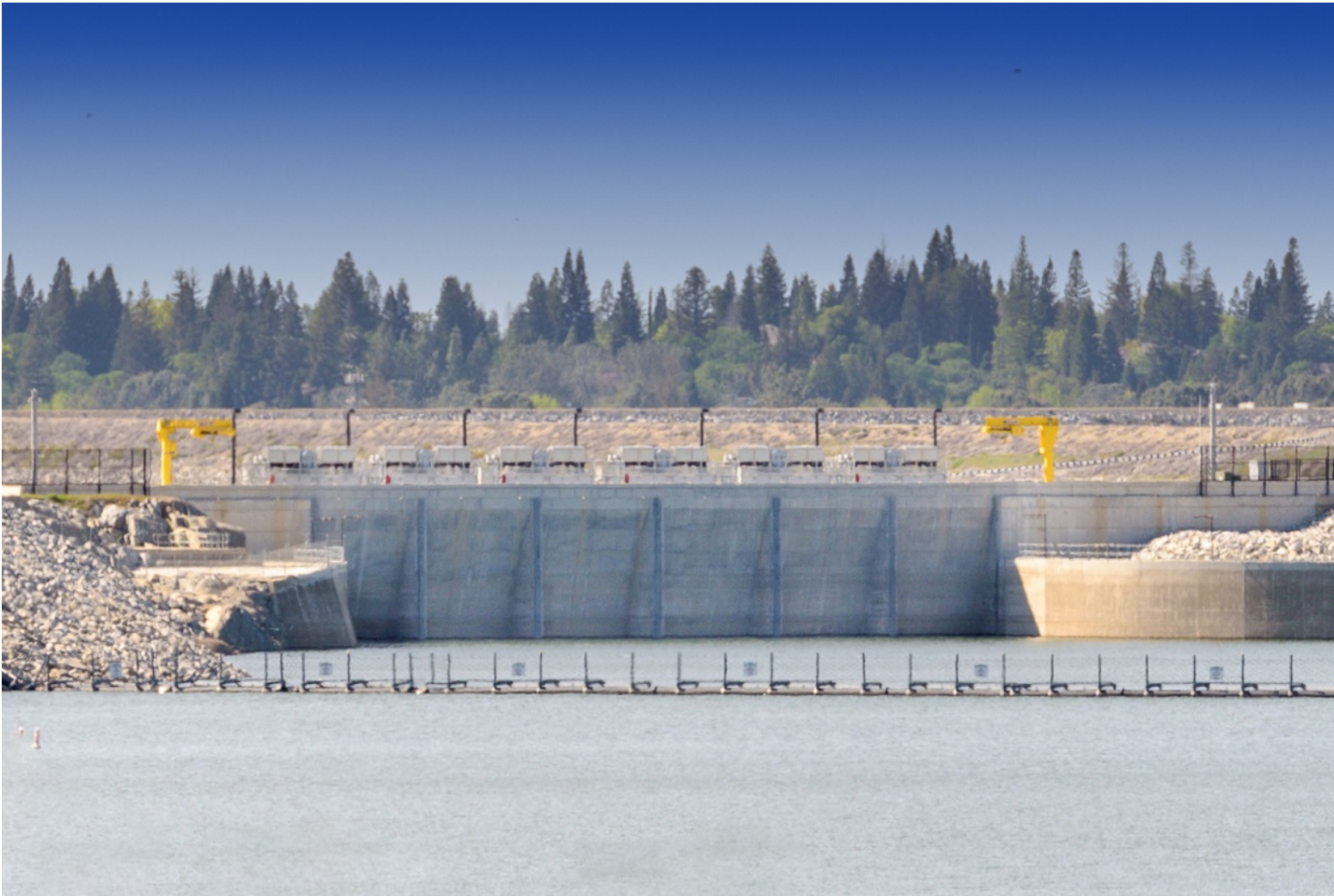
Figure 124. Auxiliary spillway for Folsom Dam (Source: image courtesy of William A. Fraser).
