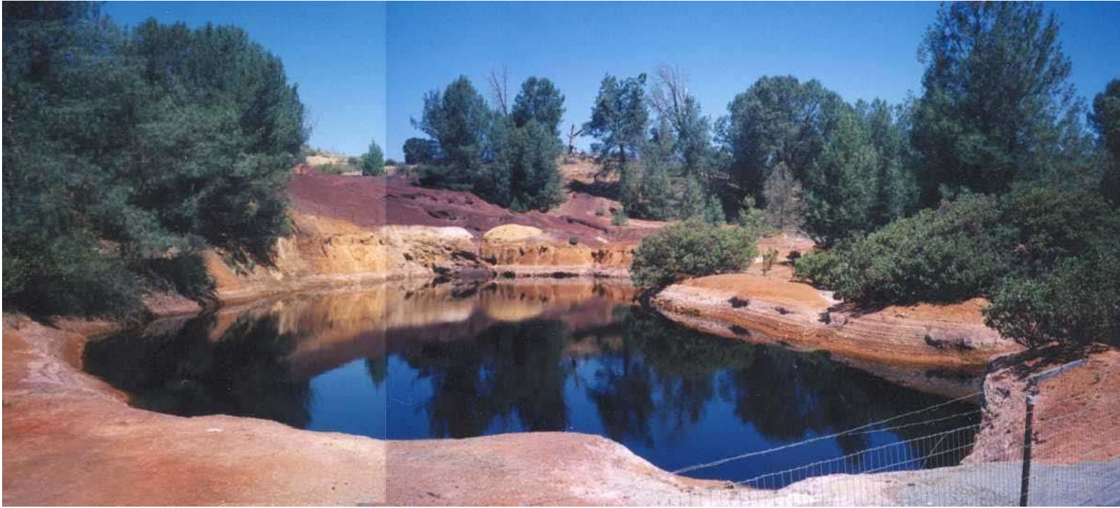
Figure 57. Image showing the 26,500 m 3 pit lake surrounded by 49,670 m 3 of acidic, heavy-metal laden mine waste (Source: image courtesy of the California Department of Conservation, Office of Mine Reclamation).
