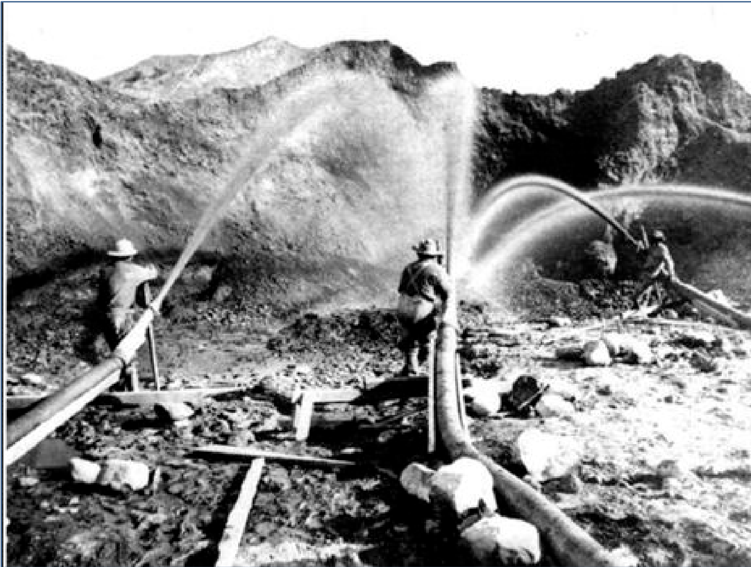
Figure 88. Hydraulic mining in California (from http://www.miningartifacts.org/California-Mines.html ).
