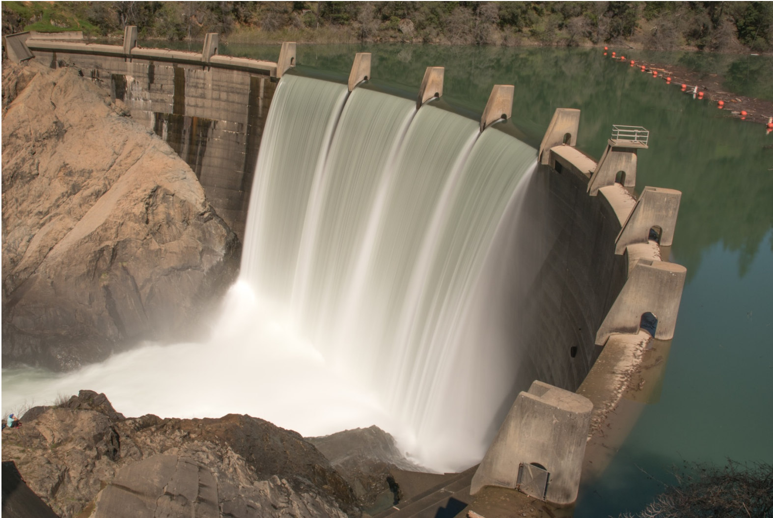
Figure 121. North Fork Dam (Source: image courtesy of William A. Fraser).
