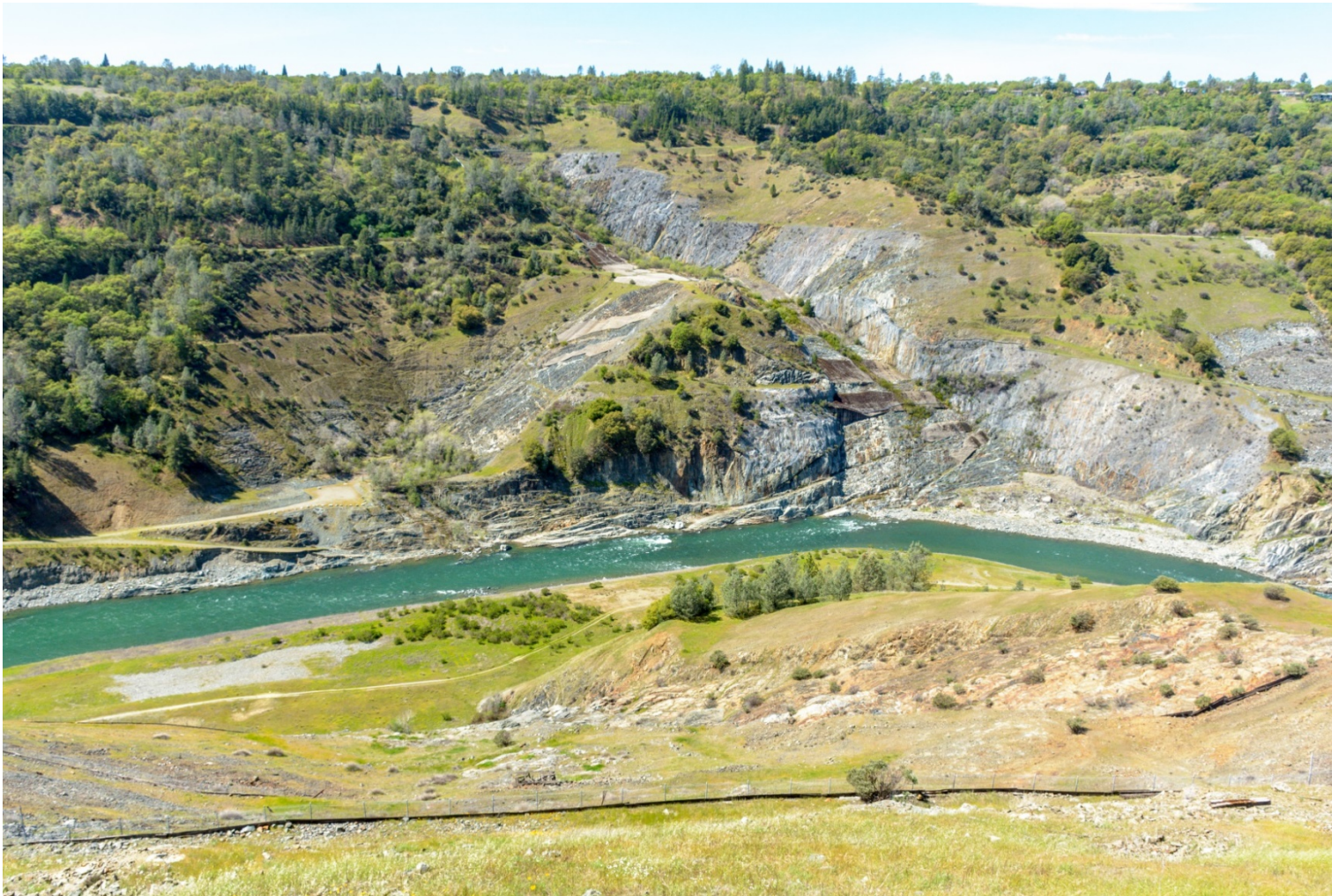
Figure 126. Auburn dam site viewed from the upper left abutment. The right abutment excavation for the arch dam and spillway channel is still visible in the landscape. The river has been restored across the dam site (Source: image courtesy of William A. Fraser).
