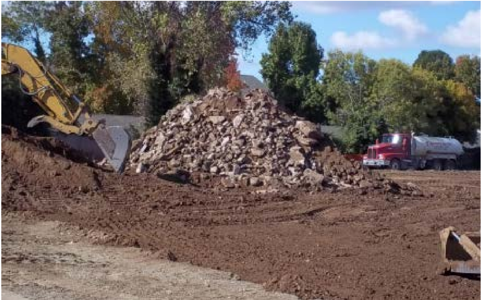
Figure 111. Photograph of typical rubble fill encountered in the Marysville, California area (Source: image courtesy of Jeremy Zorne).
