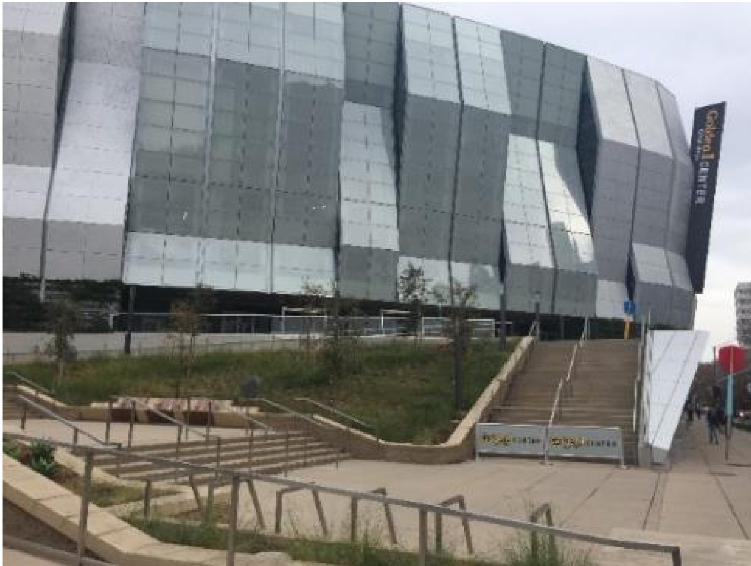
Figure 113. Photograph of Golden 1 Center during construction (Source: image courtesy of Jeremy Zorne).
