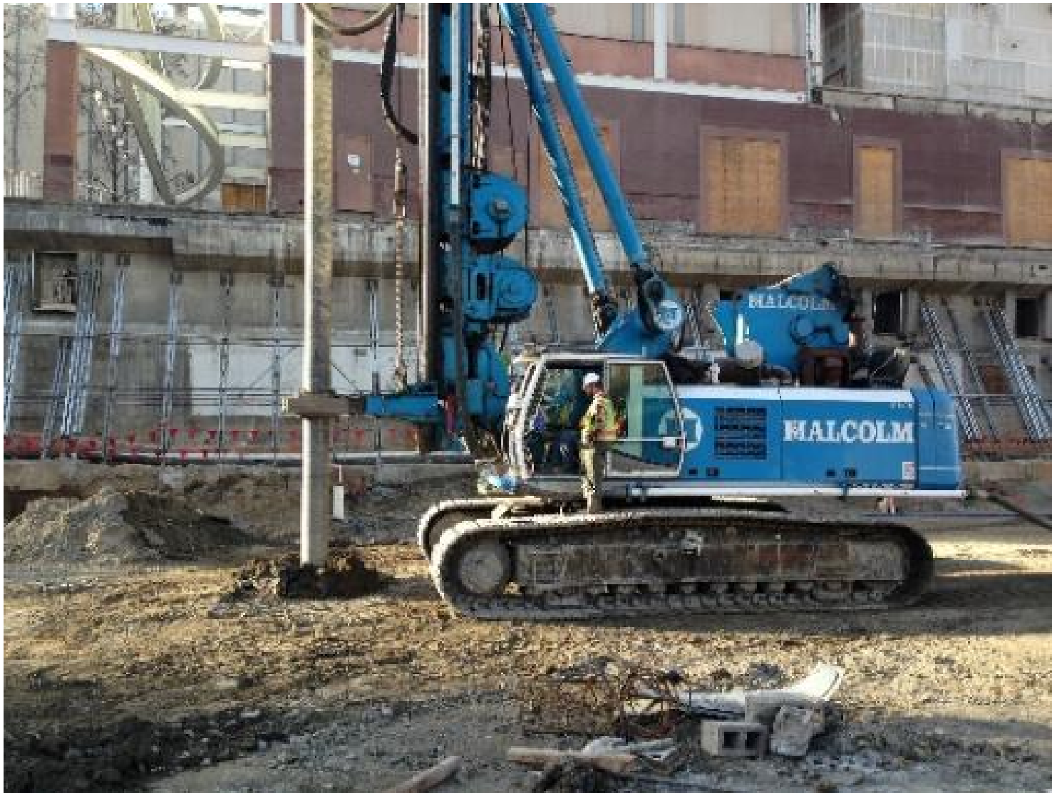
Figure 116. Displacement pile installation equipment (Source: image courtesy of Jeremy Zorne).
