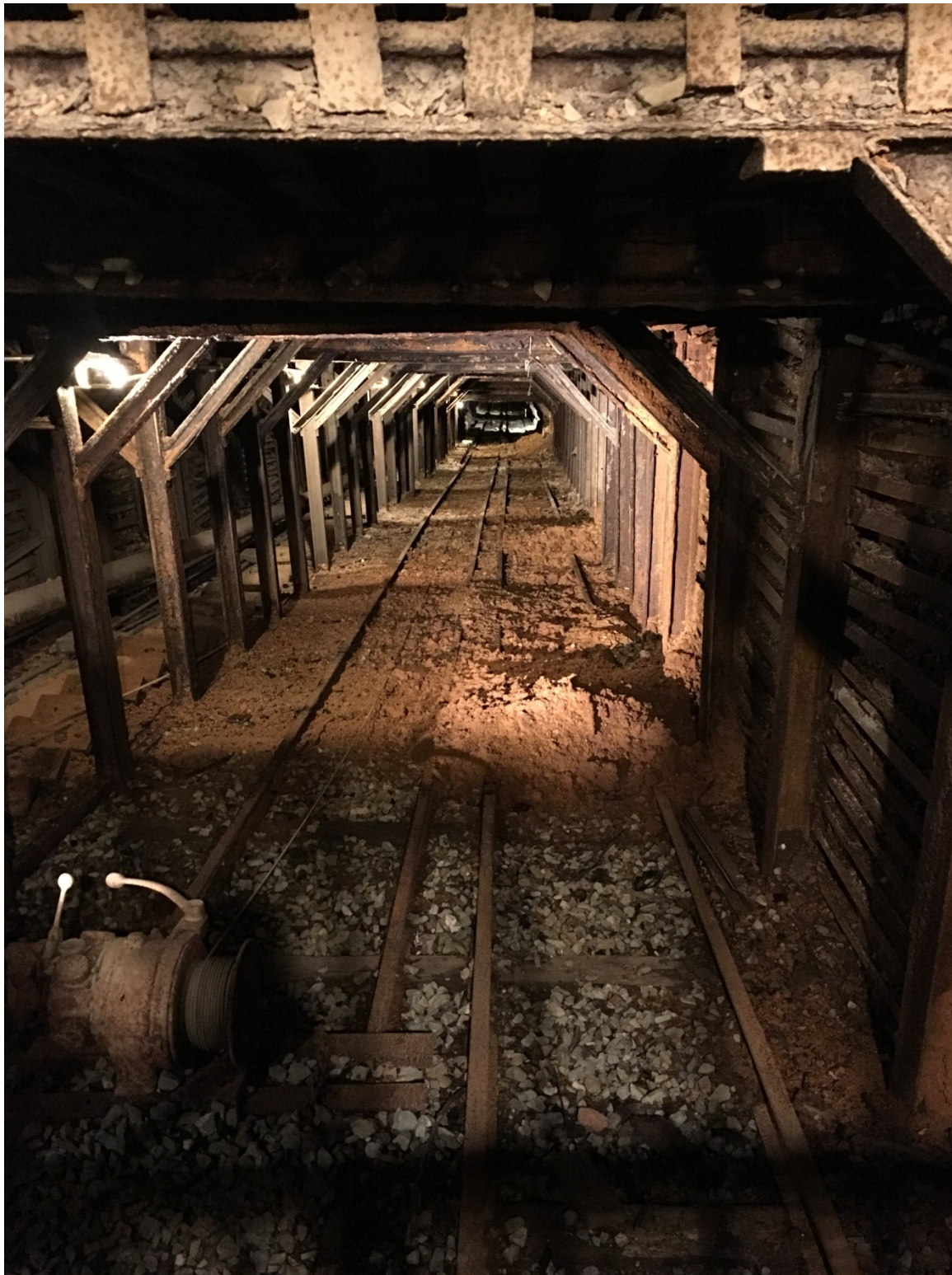
Figure 86. View down the main drift at the Empire Mine. The vein was mined by stoping with inclined shafts following dip, with horizontal shafts every 300-400 feet along strike (Stephen Testa) (Source: image courtesy of Chris Dennis).
