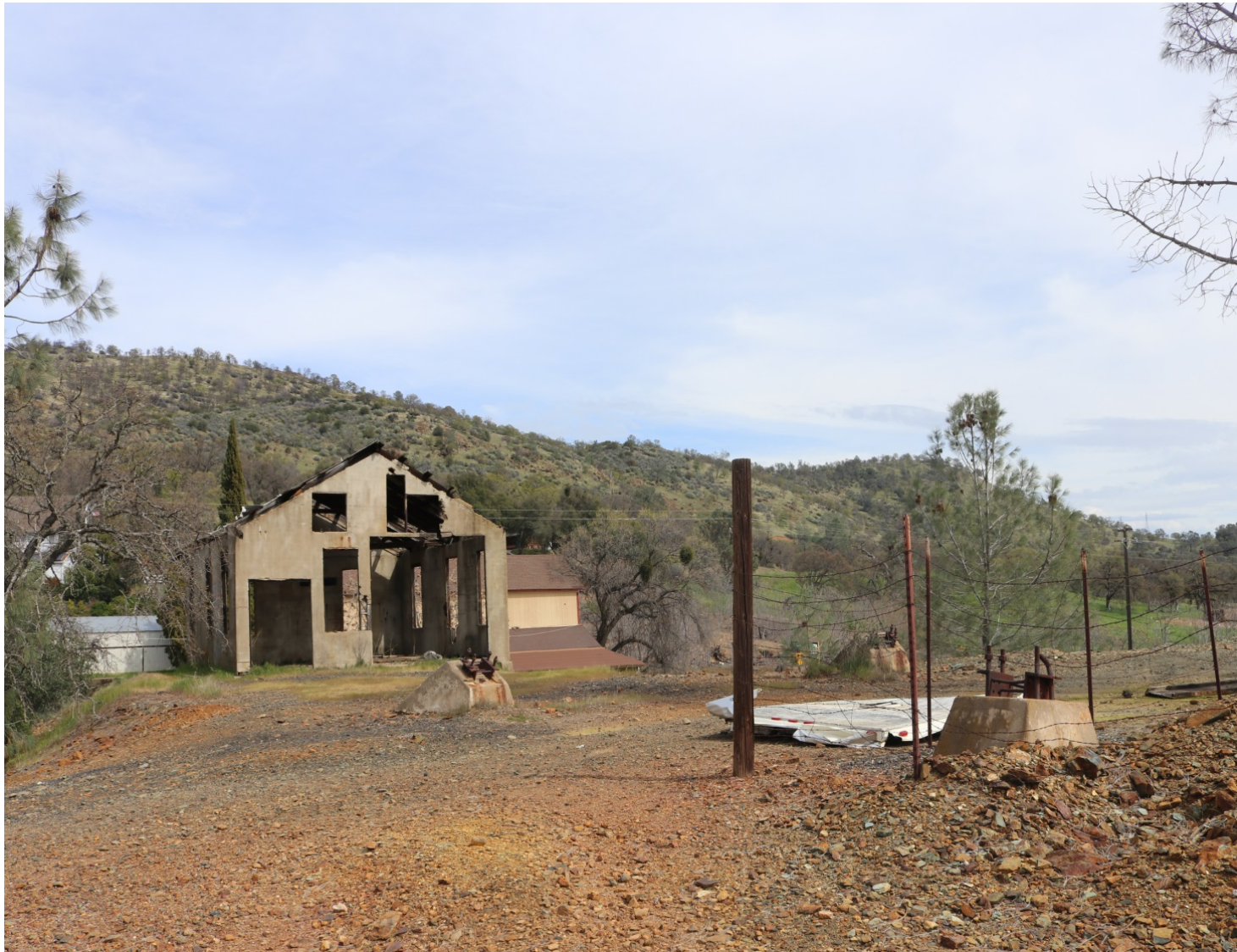
Figure 56. Surface plant of the Keystone-Union copper mine viewing southeast, with the concrete piers which held the headframe visible in foreground (Source: image courtesy of Stephen Testa).
