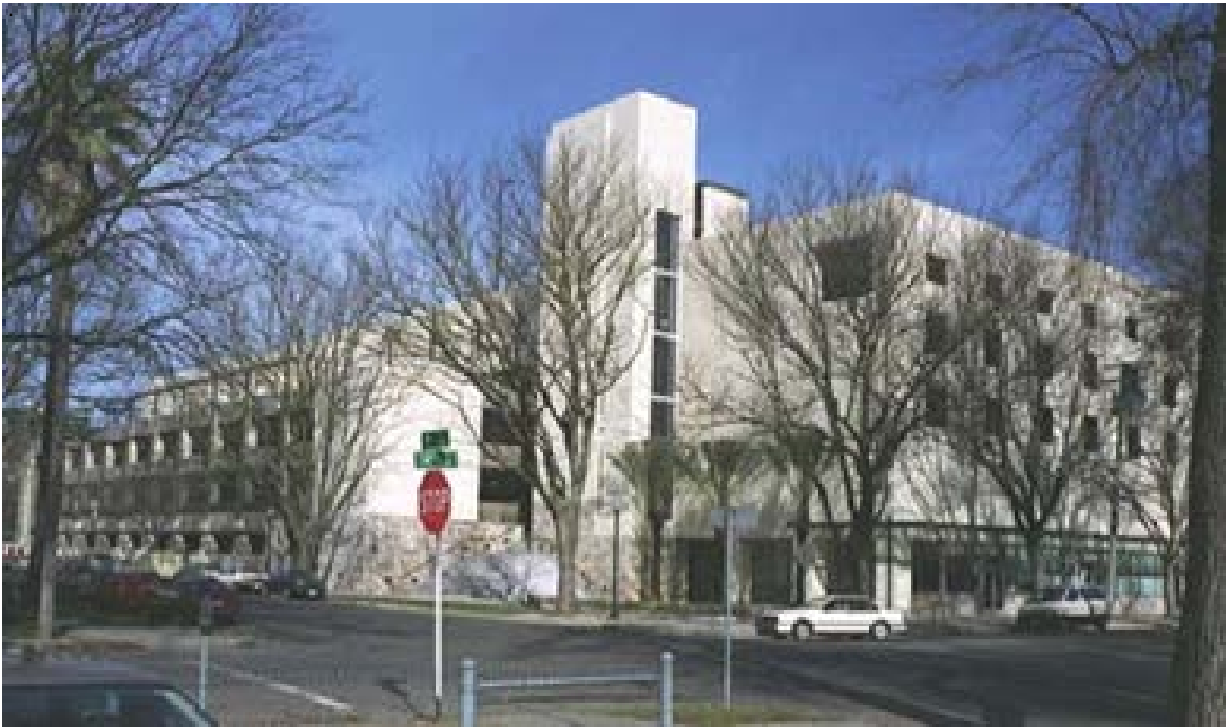
Figure 117. Photo looking northwest towards downtown parking garage and construction diagram for the parking garage (Source: image courtesy of Jonathan Manke).
