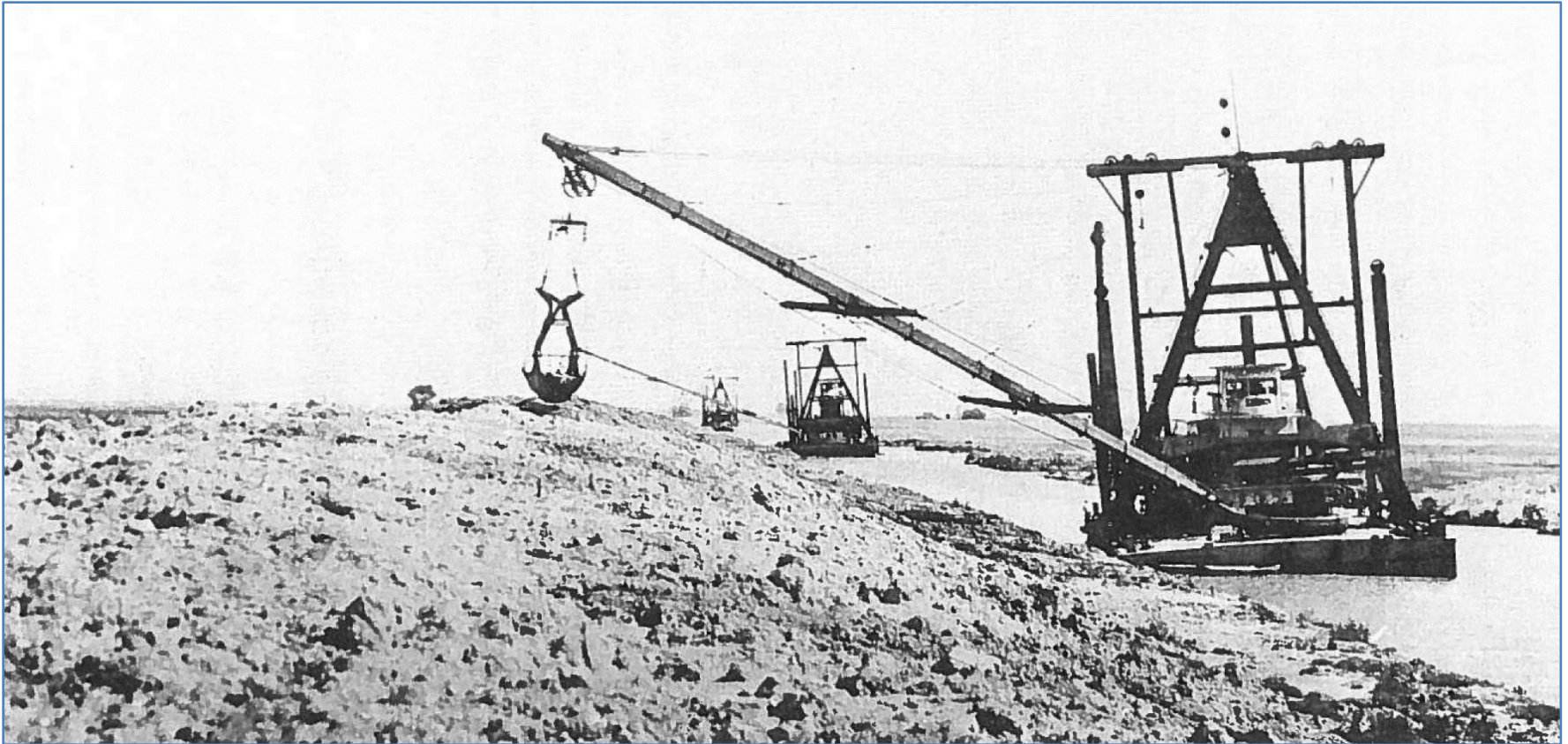
Figure 129. Clam shell dredge. Long-boom dredges constructing the east levee of the Sutter bypass (1920). The dredges progressed at a rate of about 27 m/day, ultimately emplacing 100 yd 3 of spoil per linear foot of levee. The view shows Lisbon (4.75 yd 3 , 160-ft boom), Gabilan (3 yd 3 , 182-ft boom), Argyle (4.75 yd 3 , 158-ft boom), and an unidentified dredge in the rear. (Source – California Department of Water Resources).
