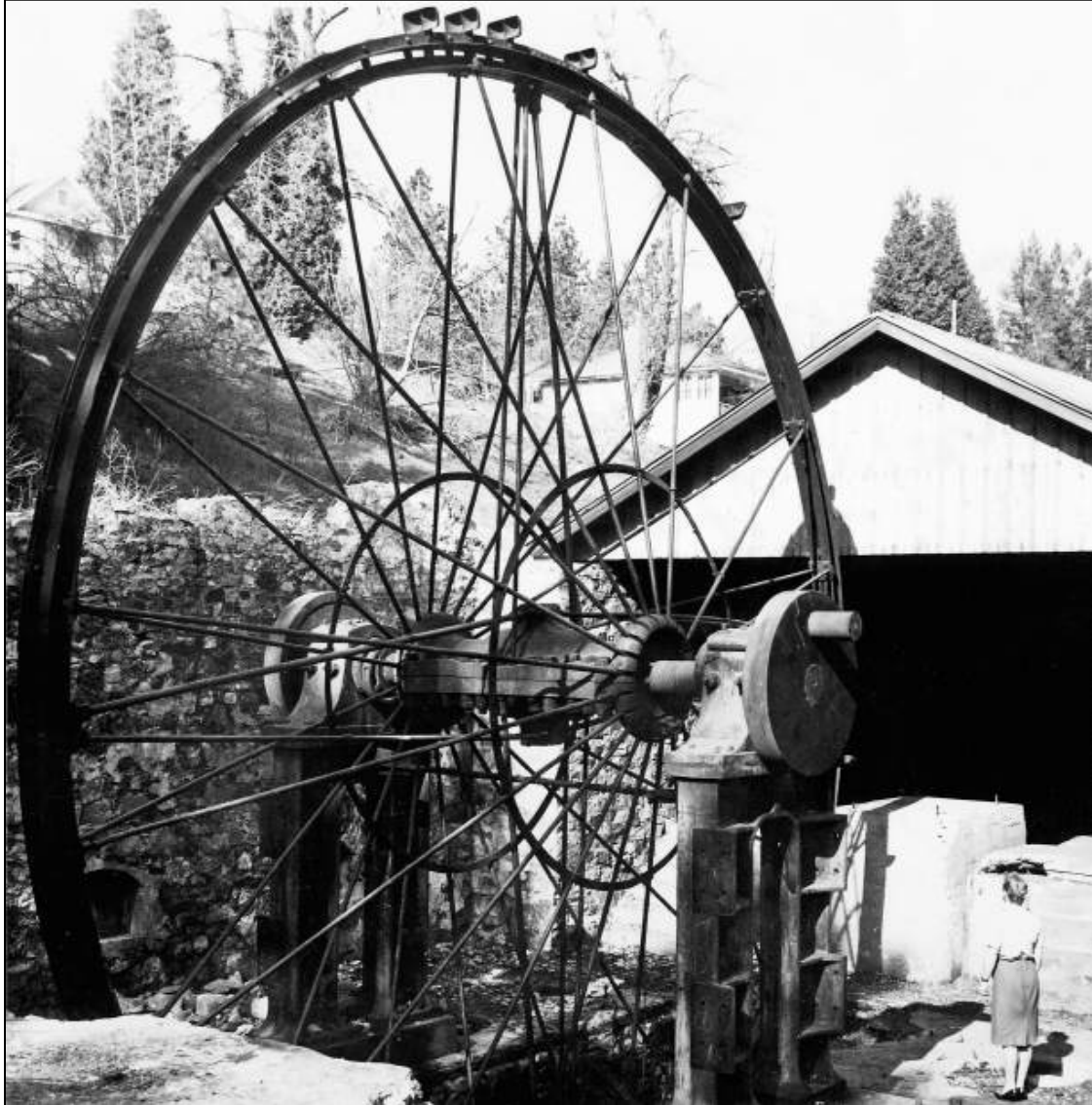
Figure 55. Pelton wheel at the North Star Mine and Powerhouse about 1950. (Source: image courtesy of The Union newspaper, Grass Valley, CA).
