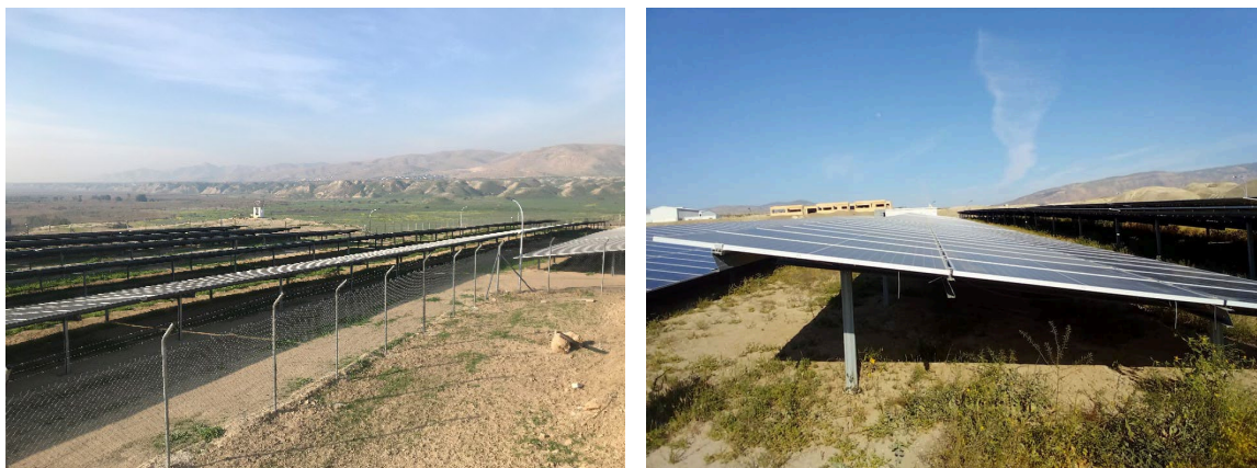
Footpaths laid out for cleaning and maintenance purposes in Deir Alla PV wheeling farm, which is a similar project that the SEED project previously delivered to Deir Alla Municipality, Jordan Valley
