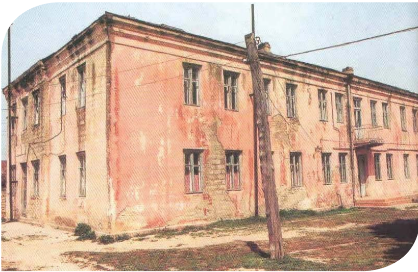
Administrative buildings of the Institute of Crop Husbandry at various times
