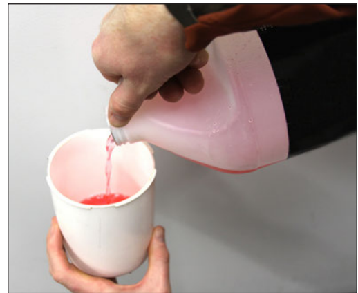
Figure 6. Pouring antifreeze from the bottle into the trap cup.
