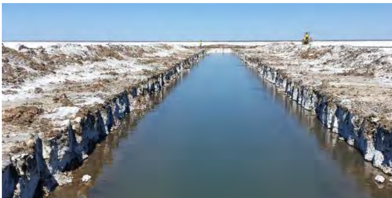
Plate 2-1: The Proposal's trial brine extraction trench
