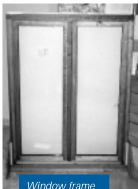
Window frame of poplar wood treated at 230°C
