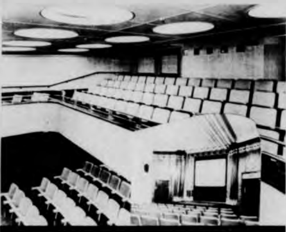
Air conditioned, 2-story Olympic Theatre
