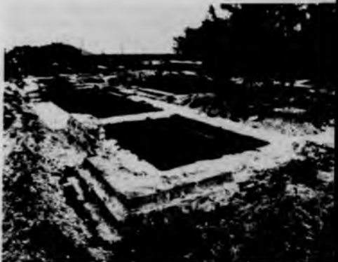
The foundation of the Turnbull Mansion on the New Smyrna, Fla. waterfront.
