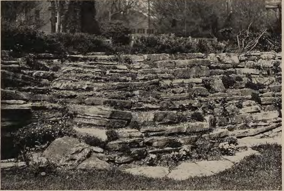
Wall Newly Rebuilt
