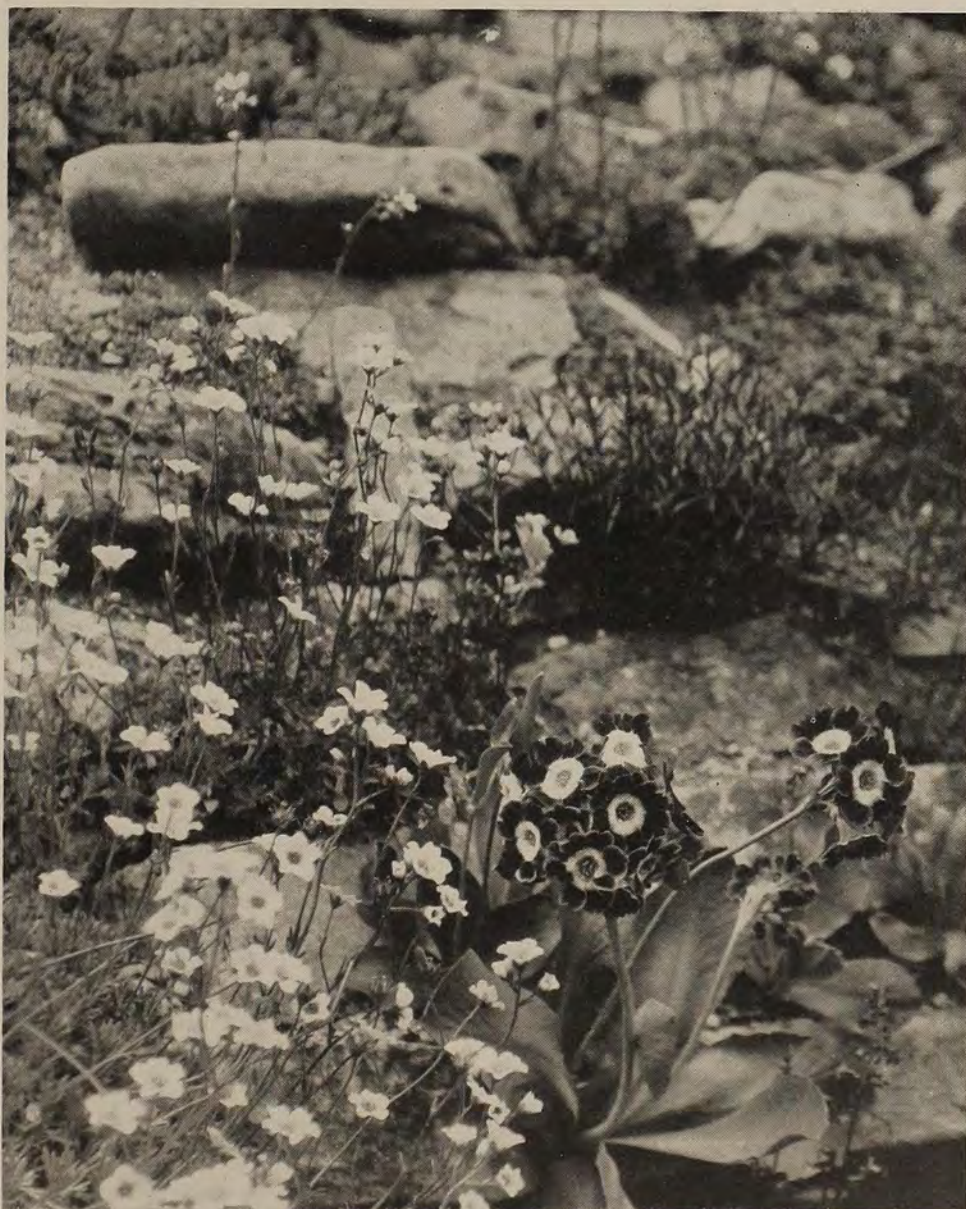
Section of wall before rebuilding showing overhanging rock which prevents plant growth beneath. Primula auricula in foreground.
