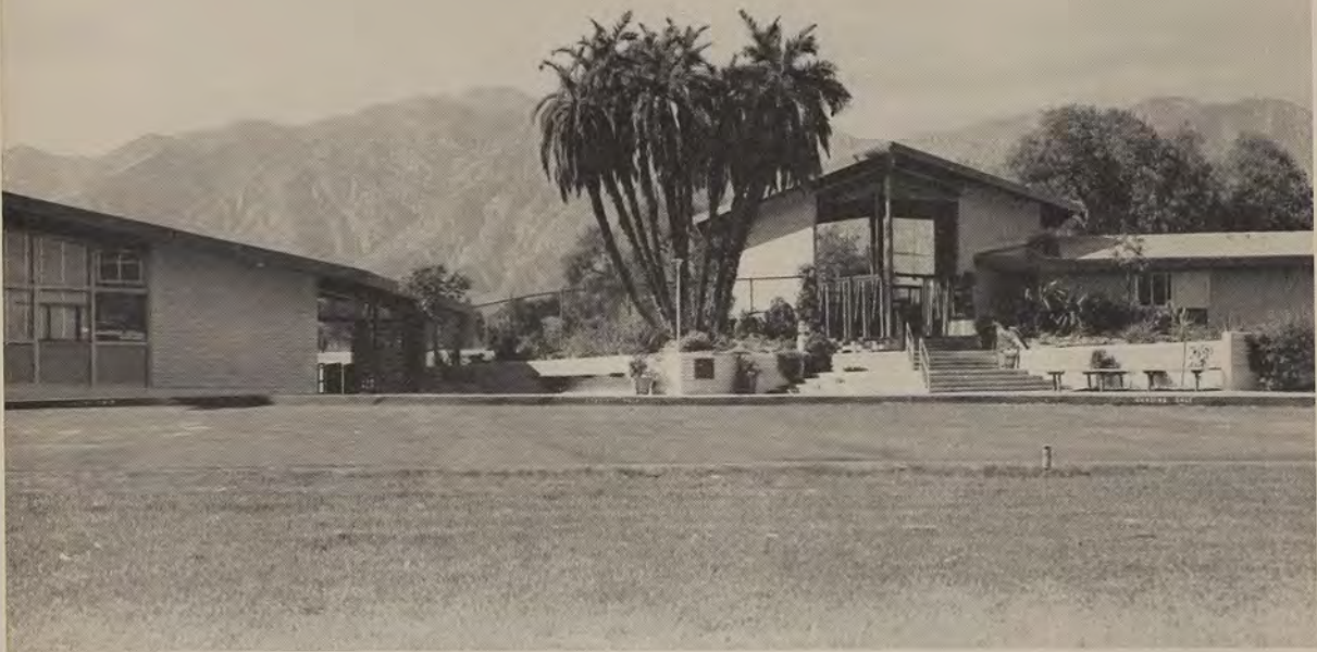
The new Arboretum administration building and gatehouse
