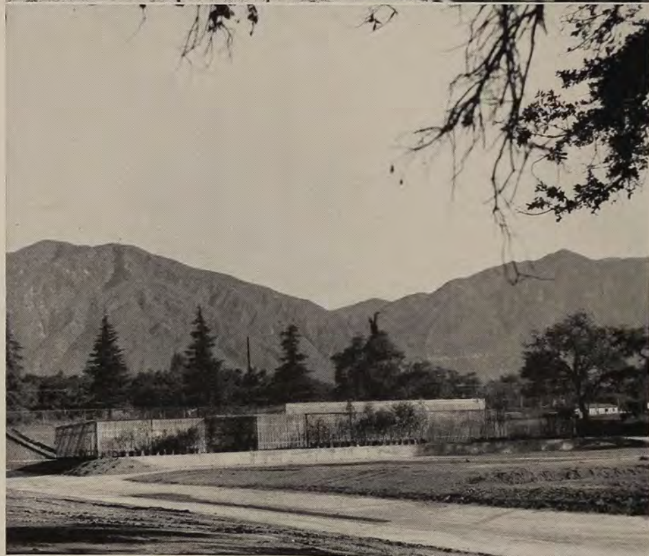
Interior and exterior views of the aluminum lath house
