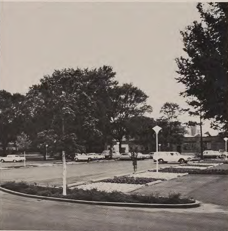
Close-up of the median strip of the deluxe lot showing drainage area, mulches, and ground cover beds under trees. Note concrete bumpers.
