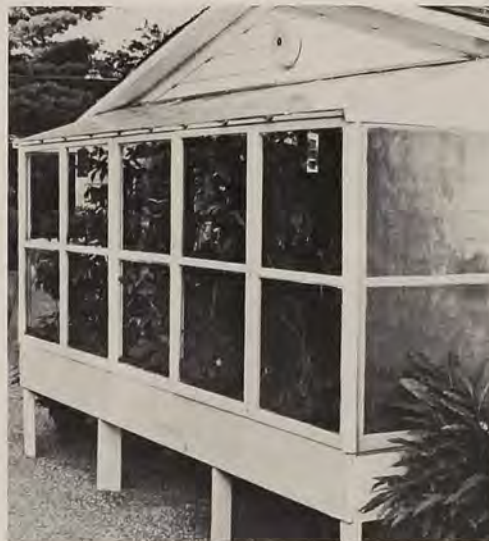
A collection of tropical economic plants were inaccessible to school groups; we built this addition for them. The plants grown in pots are imbedded in peat, so they are easy to take out for discussion. Heat circulates from three open windows in the building. For ventilation the plant windows can be opened. Glass-O-Net shades the sunny side.
