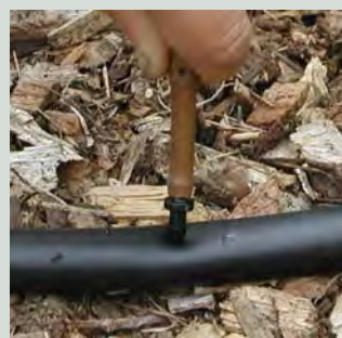
An opening is made on the header line with a hole punch, left, before it is fitted with an emitter, or dripperline, right.
