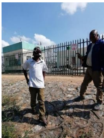
Plate 6.13 Buildings and paved areas – Dwangwa substation in the background
