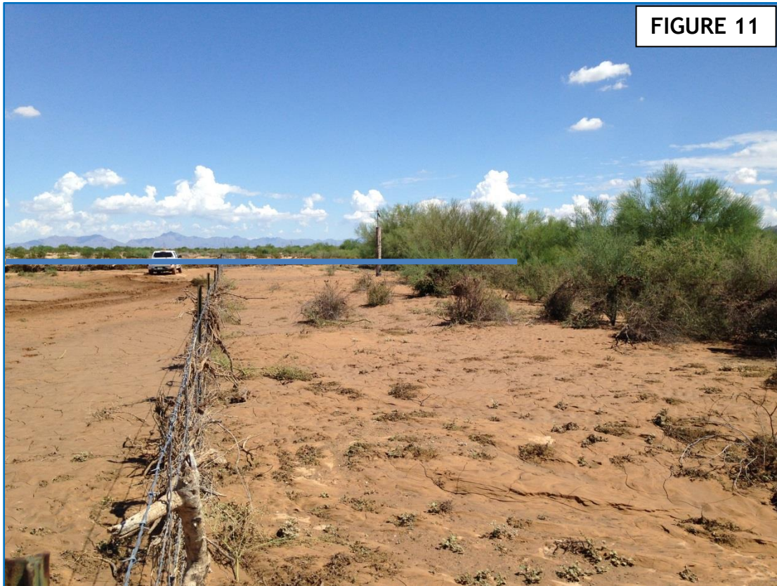
Rainbow Wash right overbank area (facing upstream), with approximate water level shown. Note debris line in fence which resulted from flow backing up at the highway culvert. (09/10/2014@13:22)
