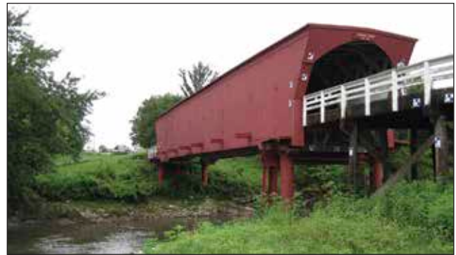
Figure 13.3—Roseman Bridge, Madison County, Iowa (2010).
