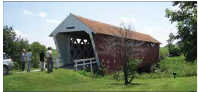
Figure 13.4—Imes Bridge, Madison County, Iowa (2010).
