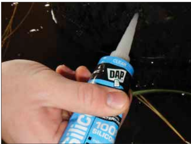
Figure 5.14—Silicone is used to fill the small drilling hole.
