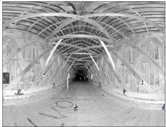
Figure 13.31—Scalar image of the inside of the Zumbrota Bridge created from a single interior scan processed with Faro Scene software.
