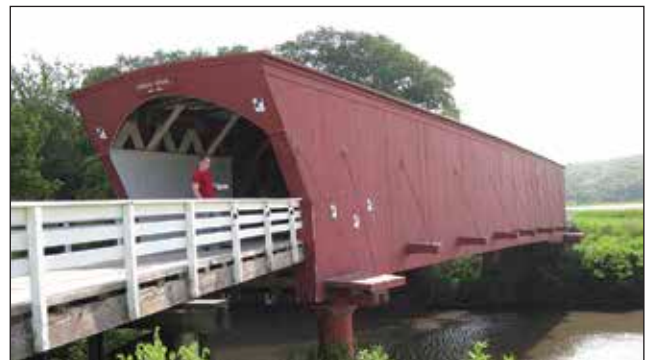
Figure 13.5—Hogback Bridge, Madison County, Iowa (2010).
