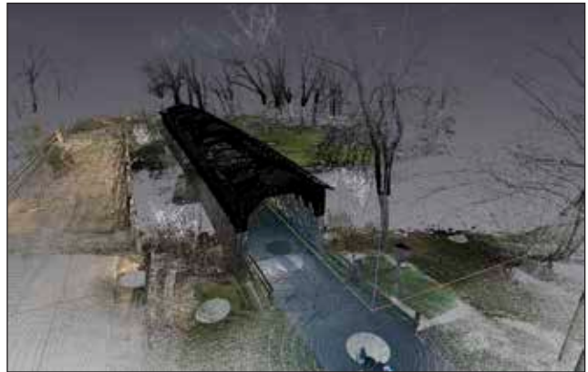
Figure 13.10—Point cloud image of the Cedarburg Bridge (SightLine, LLC).
