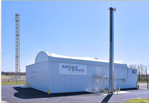
ITB Radar Facility
