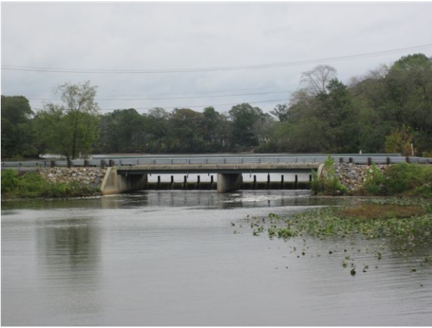
Williams Pond Dam, Seaford, Delaware, Sussex County
