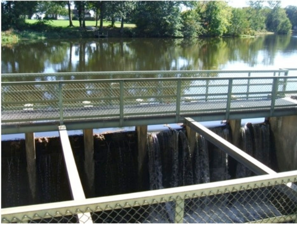
Photo 2. The spillway at Horseys Pond separating the pond from Meadow Branch looking toward the pond.
