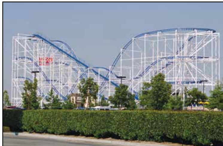
One of the largest of the Miler coasters is the Scandia Screamer in Ontario, Calif., which stands 87 feet high and has 2,600 feet of track. The coaster is currently poised for relocation. COURTESY ERIC SAKOWSKI
