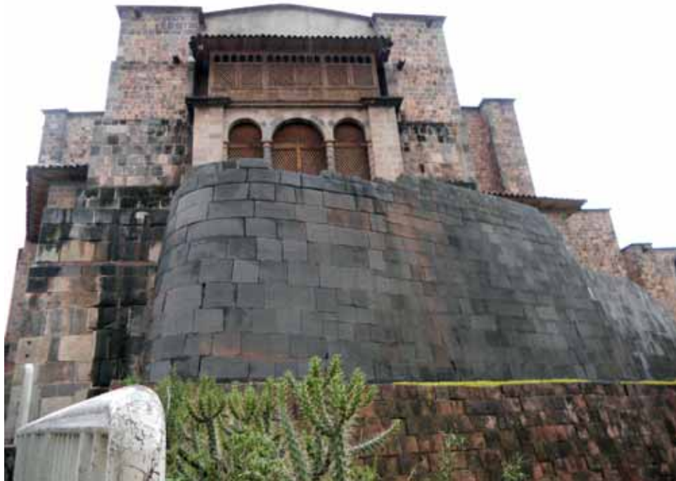
Spanish cathedral built atop Inkan walls, Qosqo City; Every time the city experiences an earthquake the cathedral collapses – the Inkan foundations never fall
