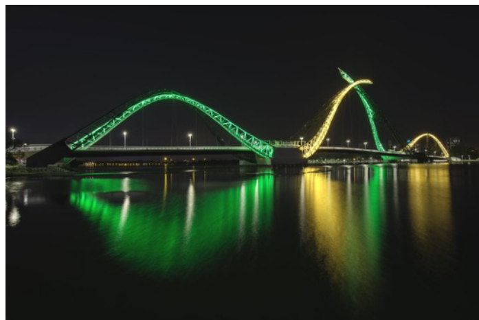
Matagarup Bridge Perth Photo: Main Roads WA
