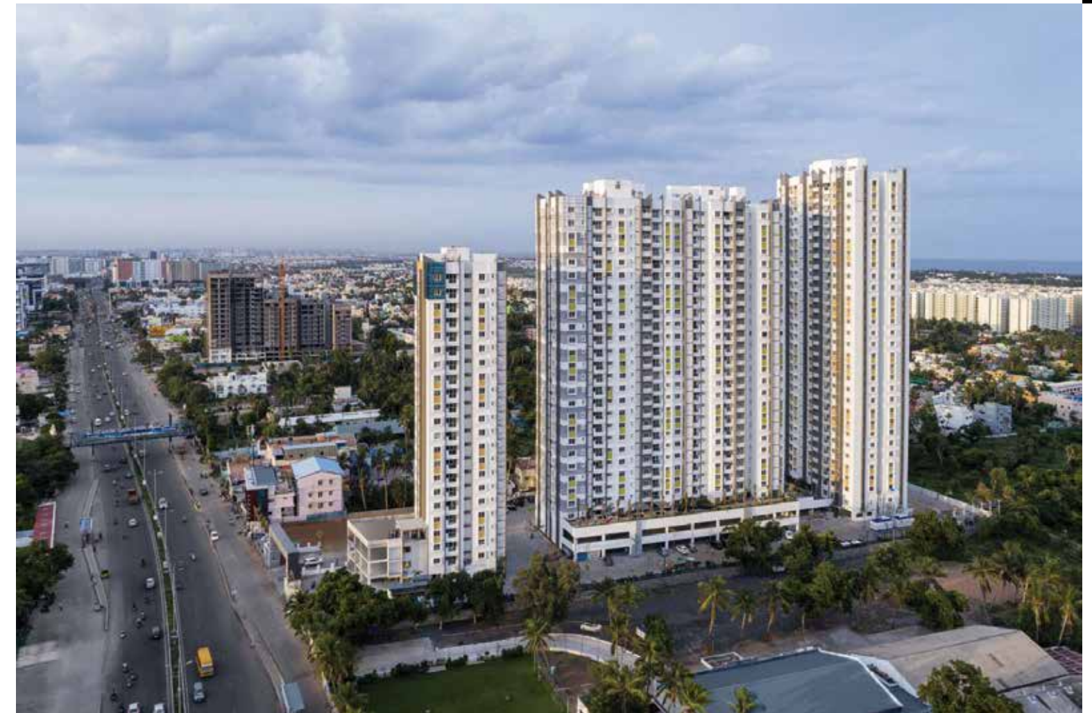
Baashyaam Pinnacle Crest, Sholinganallur, Chennai
