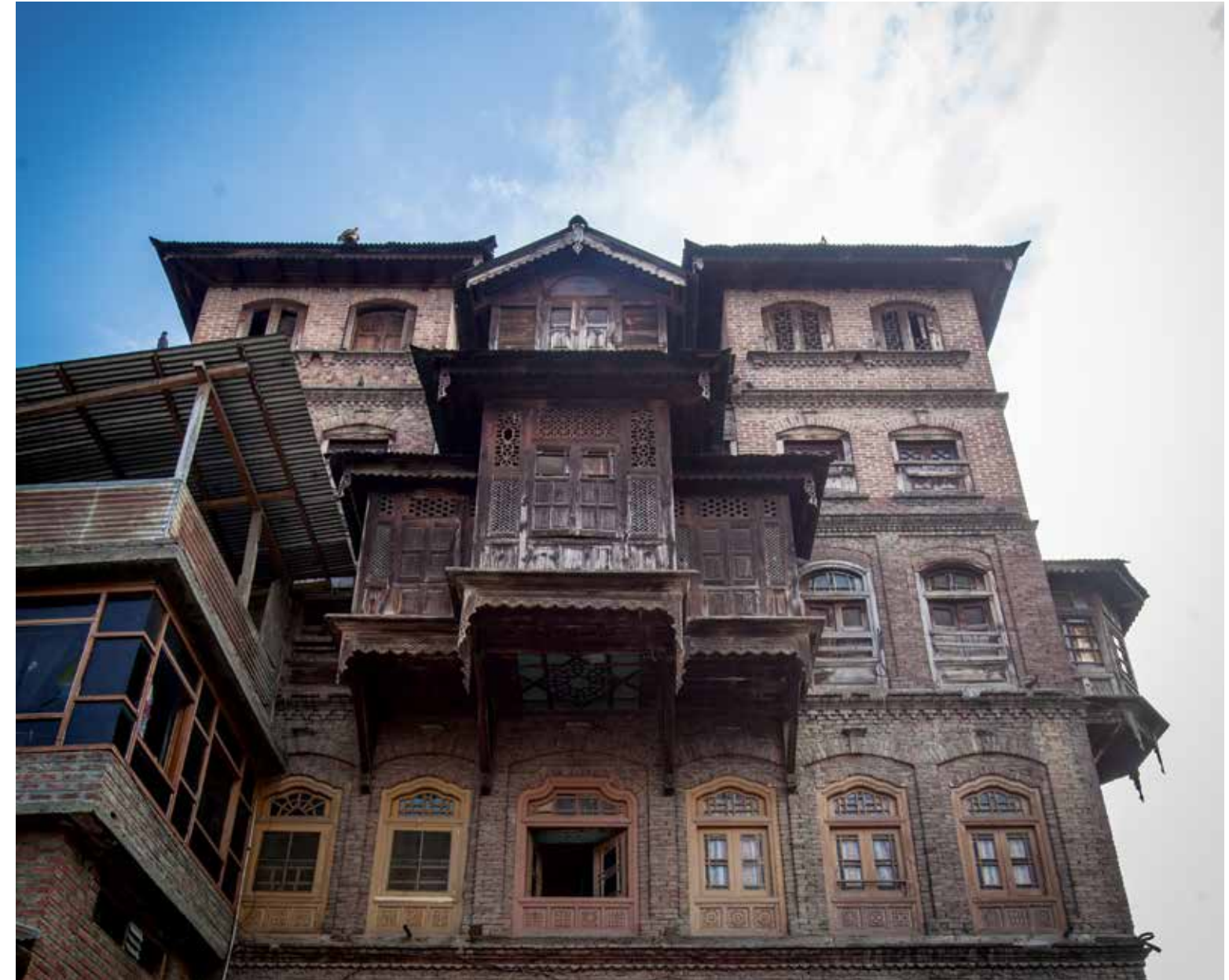
The traditional houses also mostly faced south to absorb maximum sunlight and had a single entrance along with rows of multiple windows. The wooden window frames came with small glass panes while the thick brick walls were plastered with clay and straw on the interiors to prevent the cold from seeping in.
